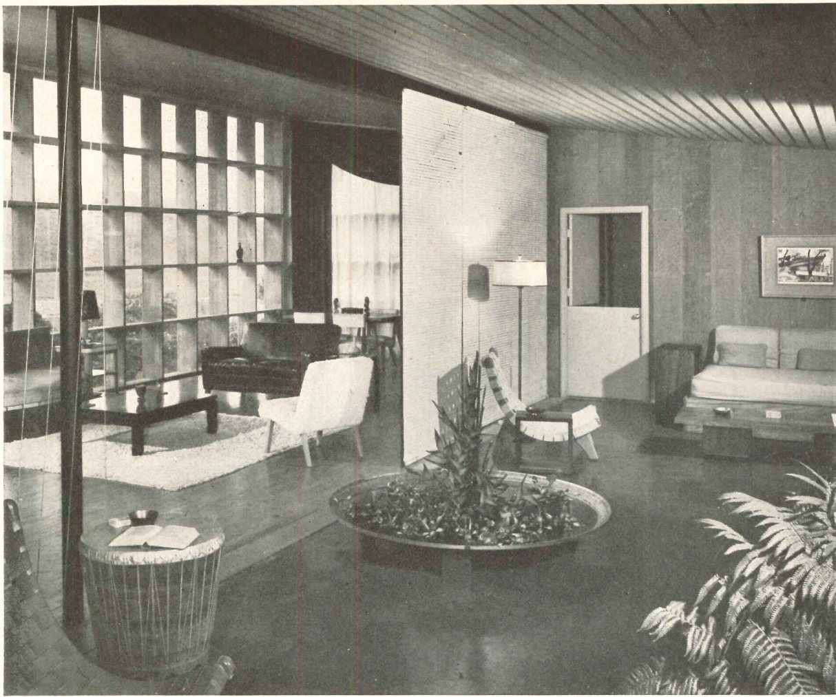
Wimberly house in Hawaii has walls of a single thickness of 1¼-in. T & G fir, like most Hawaiian houses. Floors are maple, ohia wood, and waxed green concrete. Living room and lanai (above) have a coral ceiling
