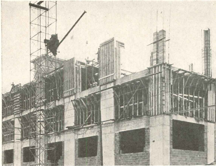
Construction shot shows erection of ventilating columns
