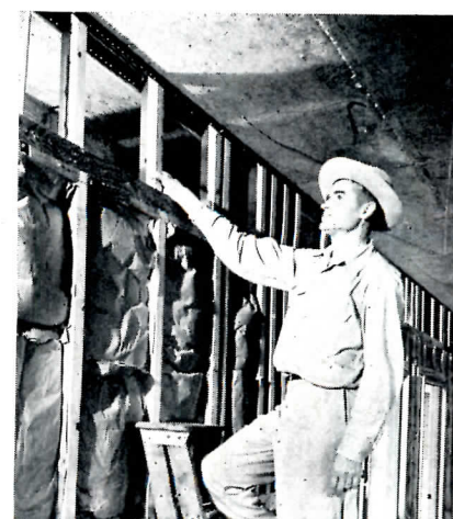
Metal runner for ceiling is installed with powder-actuated tool
