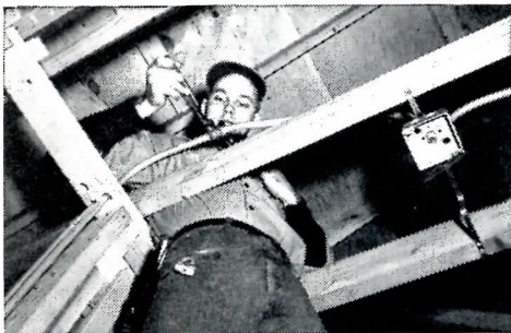
No lines to turn in close or awkward places when you're using Republic E.M.T. since every coupling is a union.
