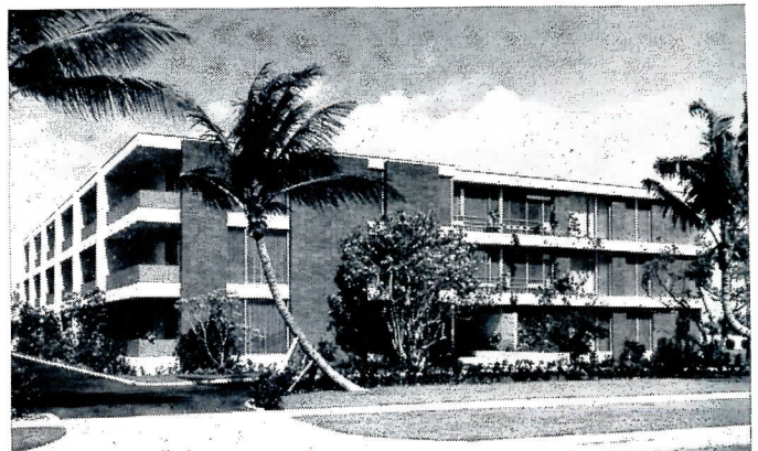
Prize winning Lanai Apartments, Miami, contains 24 units, took top honors in apartment house class in judging at A.I.A. South Atlantic Regional Conference in Miami last spring. Steeltex used only in second and third floors. Wahl Snyder, Architect. Alonzo Riley, Contractor.
