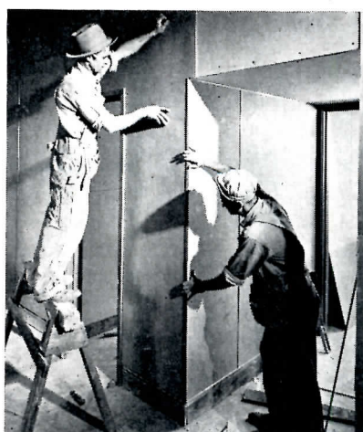
Installing cement asbestos panels over wallboard in corridor
