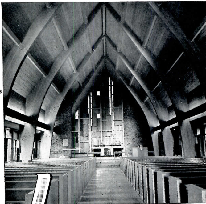
ST. LUKES LUTHERAN CHURCH MANHATTAN, KANSAS ARCHITECTS: RAMEY & HIMES WICHITA, KANSAS CONTRACTOR: GREEN CONST. CO.
