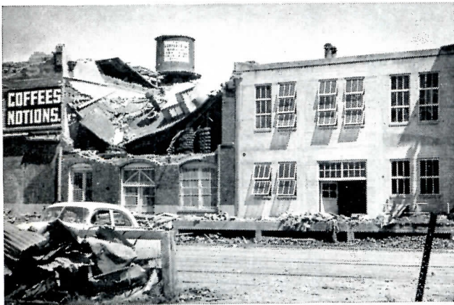
Above: Two-story building at right with reinforced concrete floors, walls and roof came through the tornado without structural damage but the adjacent structure suffered extensively. Below: This one-story warehouse was built in two sections. The section with reinforced concrete frame, floors and roof was undamaged; the other part was demolished.
