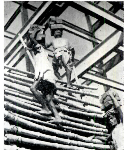
Scaffolding in Asia is most often made of strong and flexible bamboo, but is very seldom cross-braced. Workers must cling to the bamboo with their fingers and toes, for the scaffoldings are not usually equipped with foot-boards
