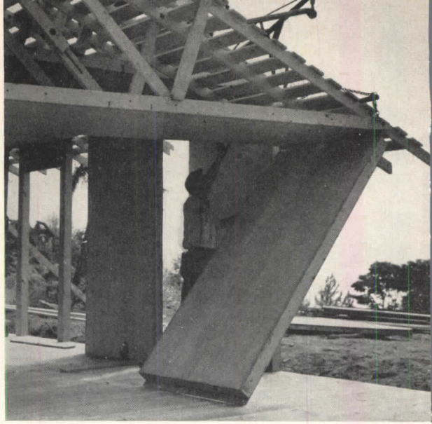
Left: Typical stressed-skin panel. Right: Stressed-skin wall panel which is hinged to ceiling panel and swings into position as roof section of three wood trusses is hoisted into position for a house designed by John Graham, Seattle architect
