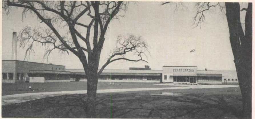
New defense factory for Lucas Rotax Ltd., Scarborough Township, Ont., is composed of four blocks: the factory itself, cafeteria block, office block and small entrance lobby. Completely air conditioned, building has minimum of exterior glass, though for psychological reasons small square windows were provided in working areas; Howard Chapman, architect
