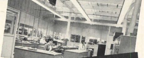
Rows of Sylvania IC Fixtures provide 50 foot candles in testing department at Sylvania's new Batavia, New York, television plant.
