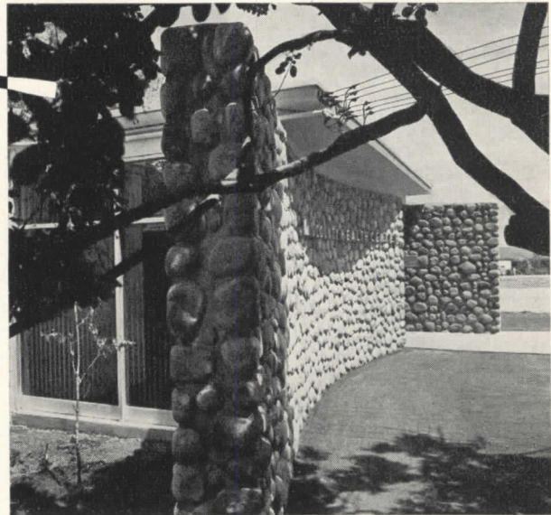
. . . are repeated on Health Center at Independence
