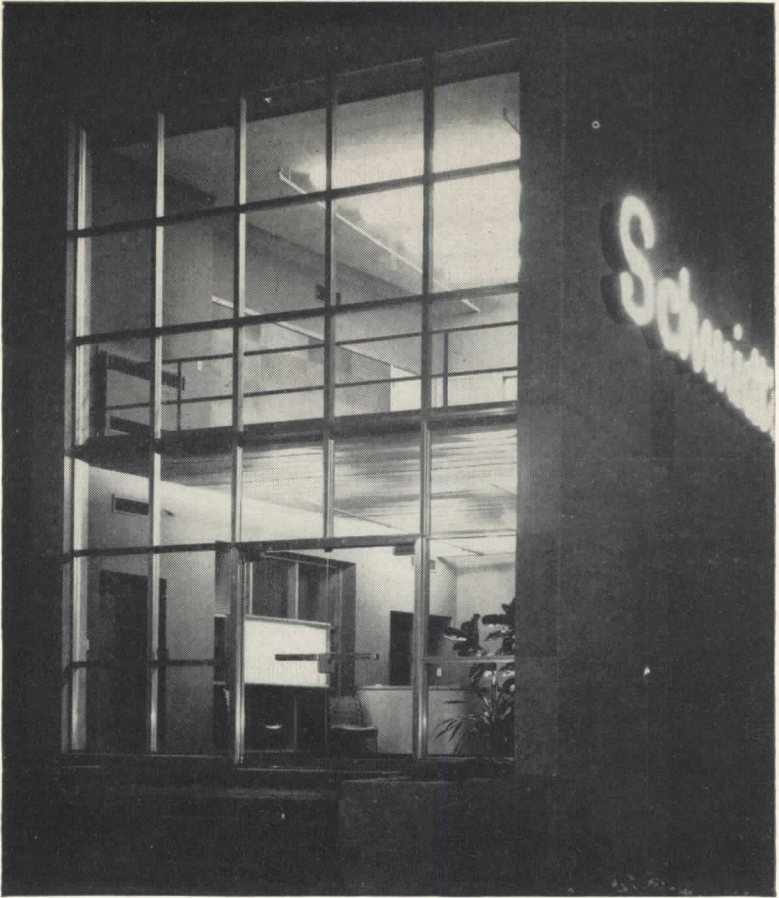
THIS INTERESTING entrance at the Schmidt Provision Company, Toledo, Ohio, is completely walled with Pittsburgh Plate Glass (approximately 20 ft. wide and 20 ft. high—running from the floor to the ceiling). It is set in Pittco De Luxe Sash No. 12 C and divided with horizontal and vertical mullions of No. 24 CTC. The doorway itself is a standard Pittsburgh Doorway, Style No. 16. Architect: Karl B. Hoke, Toledo, Ohio.
