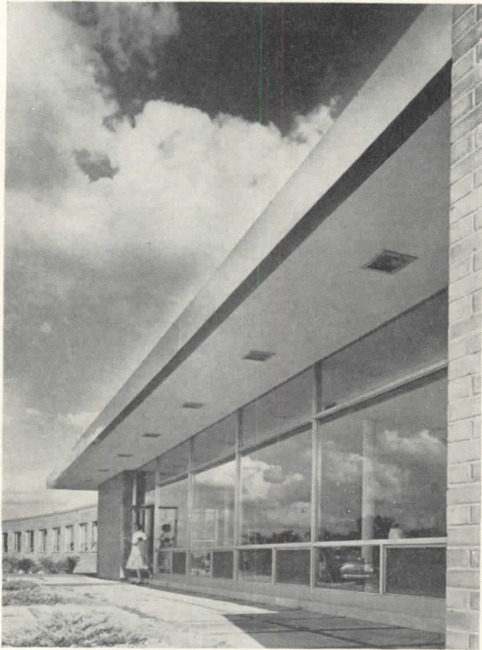
Below and right: main entrance and its lobby were kept as bright and cheerful as possible, with plenty of glass and gay modern furnishings within
