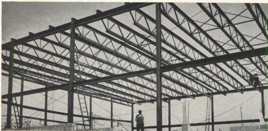
GRAND HAVEN SENIOR HIGH SCHOOL, GRAND HAVEN, MICH. ARCHITECT: WARREN S. HOLMES
