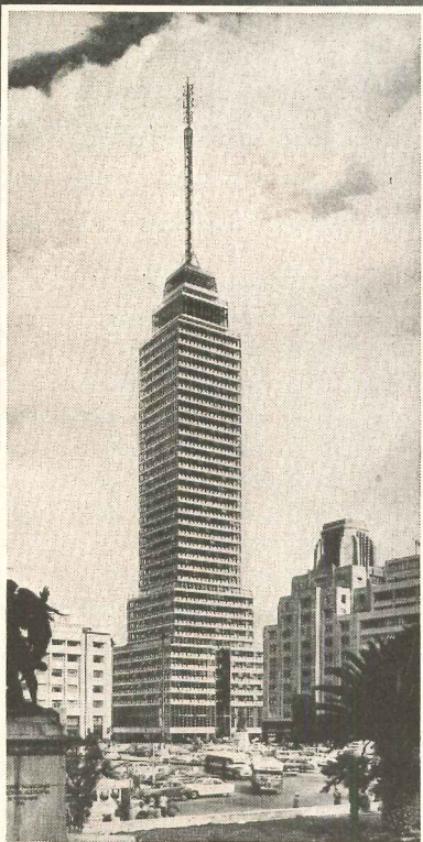
Mexico's newest and tallest skyscraper. General Director: Adolfo Zeevaert, C. E. Constructed by the Engineering Department of "La Latino Americana, Seguros de Vida, S. A." Plumbing contractor, Técnica, S. A.
