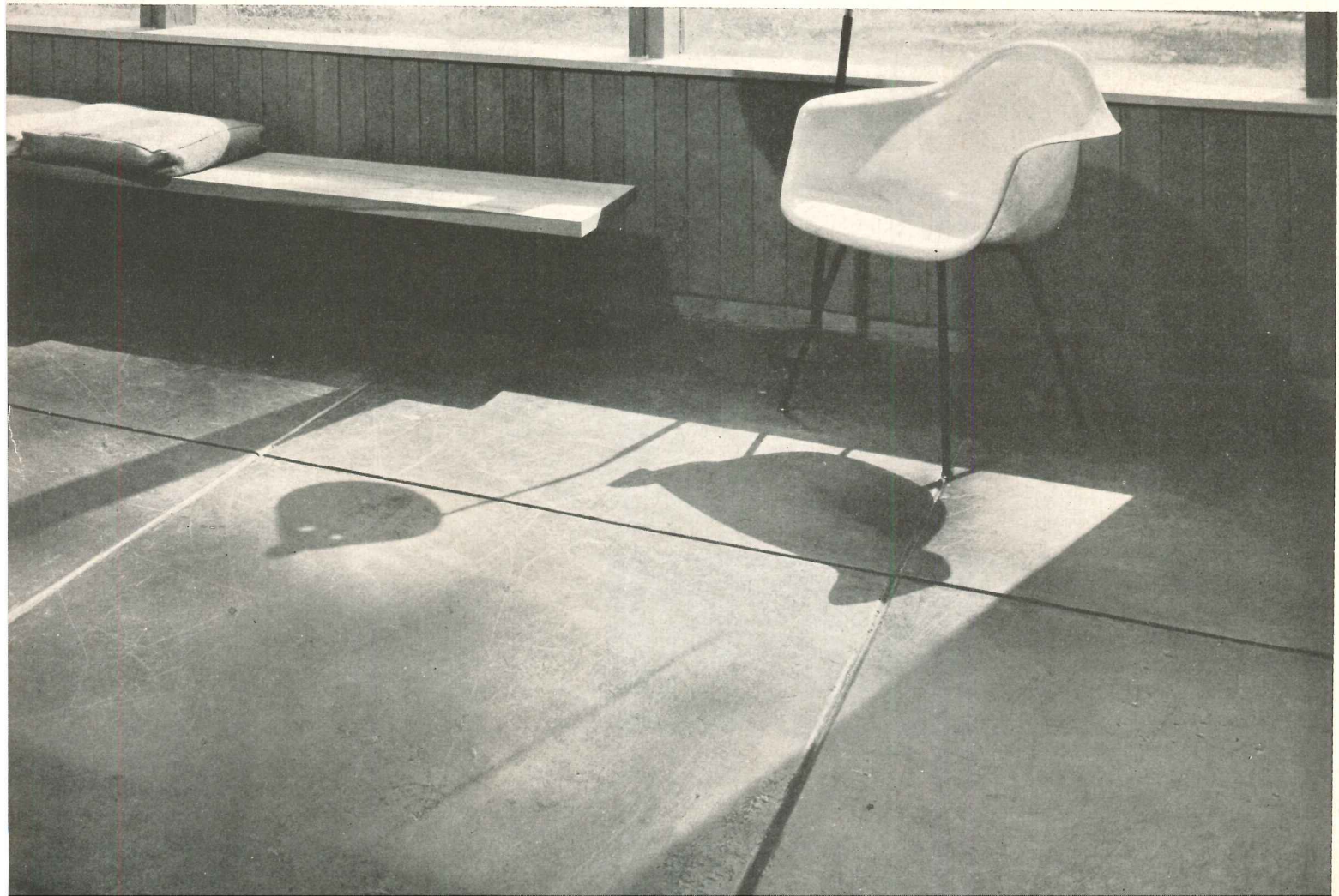
Large squares of slate: George Fred Keck - William Keck, architects. Hedrich-Blessing photo
