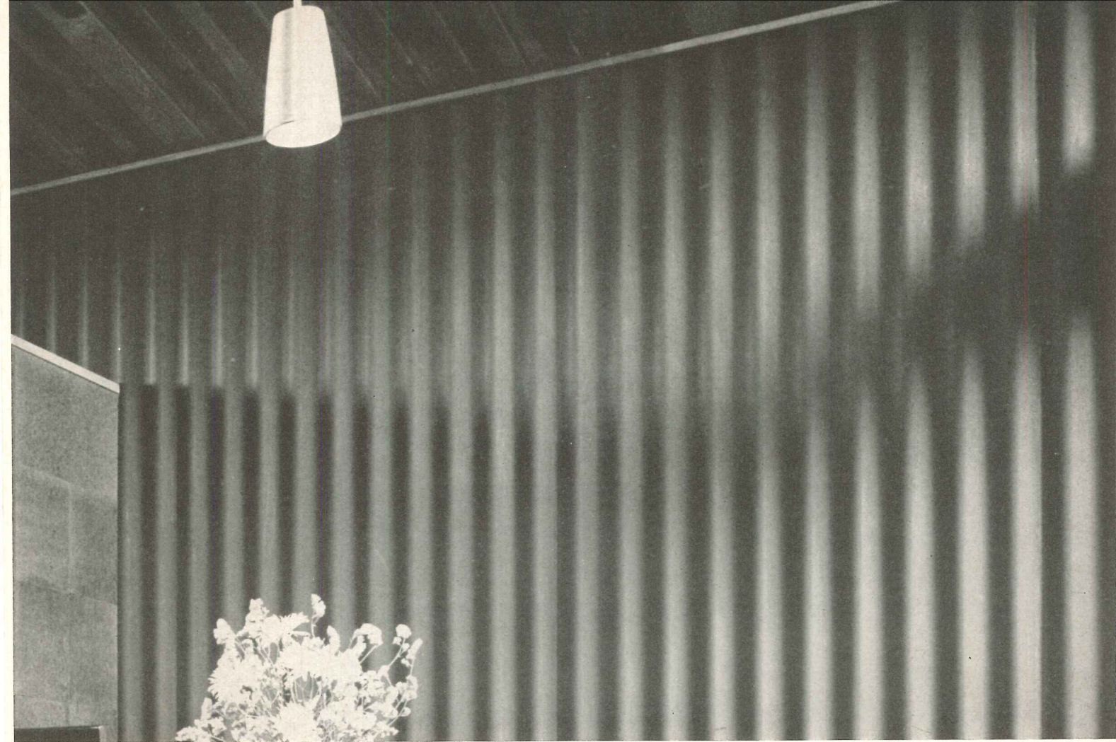
Corrugated asbestos sheeting on wall: Curtis & Davis, architects. Joseph W. Molitor photo
