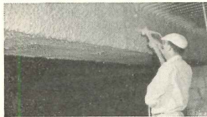
Prudential Building. Zonolite Plaster machine-applied to beams for fireproofing.
