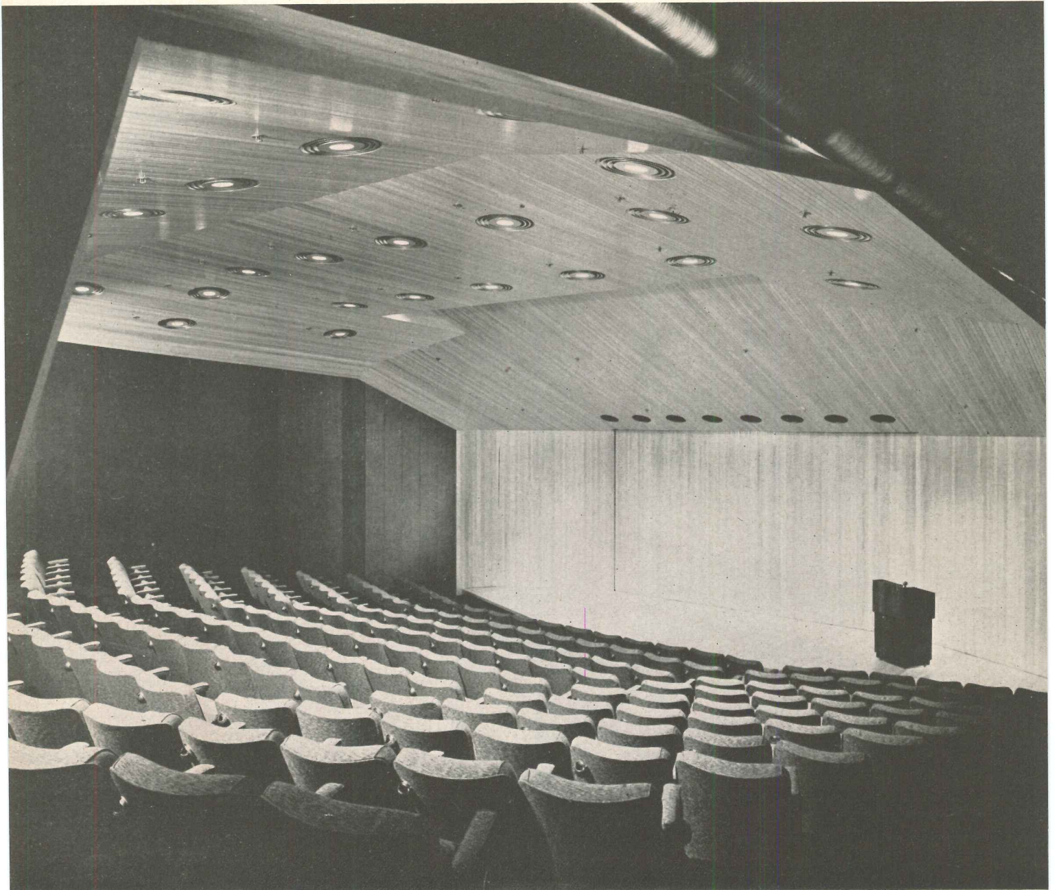
Auditorium, Process Development Administration Building
