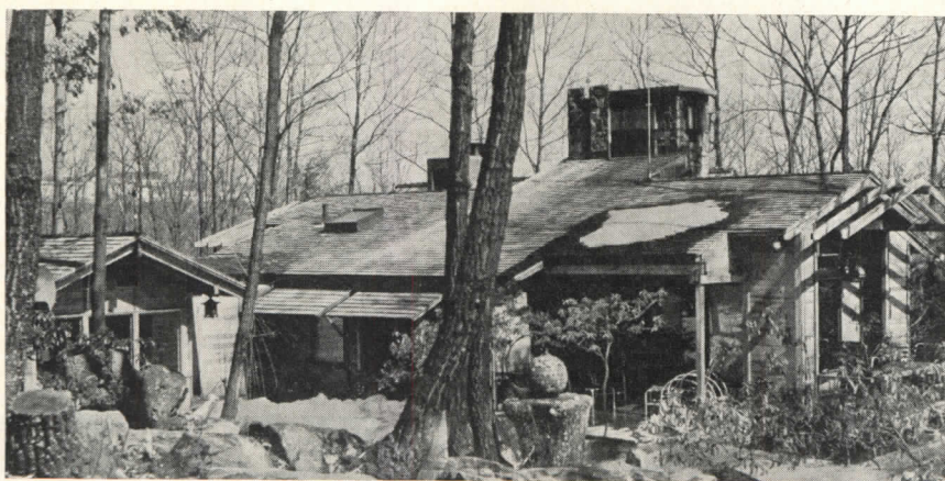
SLIDING SHUTTERS (above) is the Harwell Harris-designed residence of a New York stockbroker who has announced plans to subdivide part of his estate in Redding, Conn., into ten large sites for houses with the specified purpose of establishing a show-place of contemporary architecture. Gerald M. Loeb, a partner of E. F. Hutton & Co., plans to consult with early purchasers of the sites — they must also be devotees of distinctive architecture — to compile a roster of architects for the houses; but he mentions such names as Frank Lloyd Wright, Harwell Harris, Philip Johnson, Richard Neutra, Marcel Breuer, Paul Rudolph, John Johanson, Edward Barnes, Hy Hebeln, Raphael Soriano, Charles Eames and Bruce Heiser
