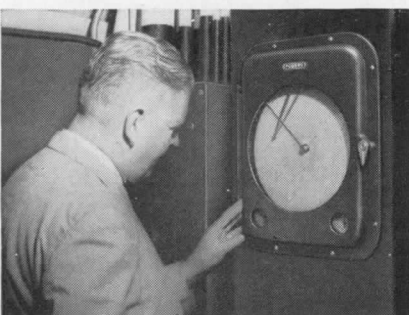
Below: Powers Recording controller regulates temperature of chilled water used for comfort air conditioning.
