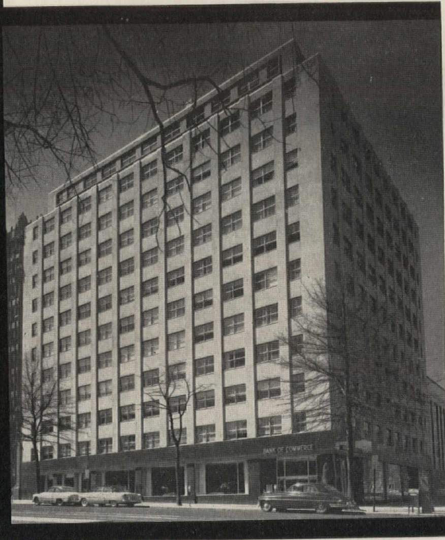
Bank of Commerce, Washington, D.C. Here's an example of concrete joist construction through use of Ceco Steelforms. Concrete was reinforced with Ceco Rebars. Ceco 200-B Aluminum Double-Hung Windows provide adequate daylighting and weathertight protection. Architect: Corning & Moore; Contractor: Standard Construction Company, Inc.
