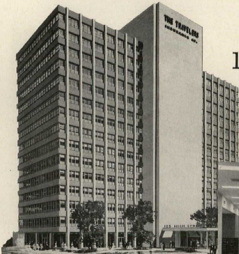
Architects: Kahn & Jacobs, New York City Consulting Engineer: Jaros, Baum & Bolles, New York City General Contractor: George A. Fuller Co., Boston, Mass. Electrical Contractor: Lord Electric Co., Boston, Mass. Electrical Distributor: George H. Wahn Co., Boston, Mass.
