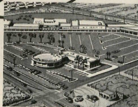
Shoppers Haven Shopping Center, Pompano, Fla. Zonolite concrete over galvanized steel deck. Roof area, 120,000 sq. ft. William Vaughn, Arch., DeBritt & Assoc. Engr. Roof deck sub-contractor: Commercial Roof Decks, Inc.
