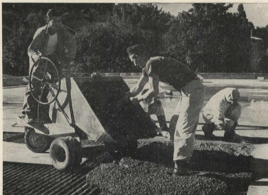
Pouring is no problem with Fab-Form. Here a buggy has rolled over Fab-Form without damaging the material. Six-inch square mesh made of No. 6 gage wire is from Pittsburgh Steel, too.
