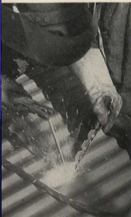
Exclusive Fab-Form Welding Washer Stick reduces installation time. After the end washer on the stick is bent up, the welder makes a plug weld and snaps off the washer. Then mesh is installed and slab is poured.
