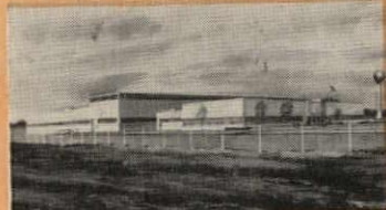
CUTLER-HAMMER, INC. Lincoln, Ill. Designer-Engineer-Builders: The Austin Company, Cleveland Plumbing Contractor: J. F. Weiskopf & Son, Springfield, Ill.
