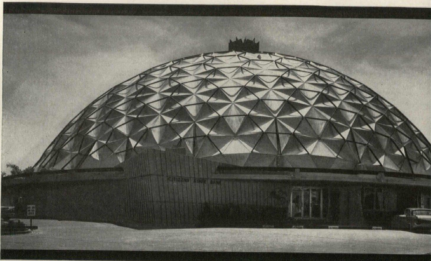
Citizens State Bank, Oklahoma City, Oklahoma. Three Ceco products were used to help achieve a dramatic architectural effect here. The products were Reinforcing Steel, Wire Mesh and Open-Web Steel Joists. Architect: Bailey-Bozalis-Dickson and Roloff; Contractor: Secor Building Company, Incorporated.
