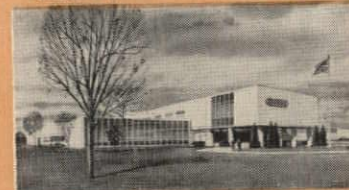
CHARLES BRUNING COMPANY, INC. Mt. Prospect, Ill. Engineer-Architect: A. Epstein & Sons, Inc., Chicago Plumbing Contractor: Marcus Weil & Sons, Chicago
