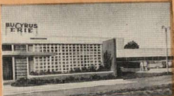
BUCYRUS-ERIE COMPANY Richmond, Ind. Designer-Engineer-Builders: The H. K. Ferguson Company, Inc., Cleveland
