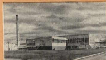
KAISER ALUMINUM & CHEMICAL COMPANY, Ravenswood, W. Va. Engineer-Designer: Kaiser Engineers, Division of Henry J. Kaiser Company
