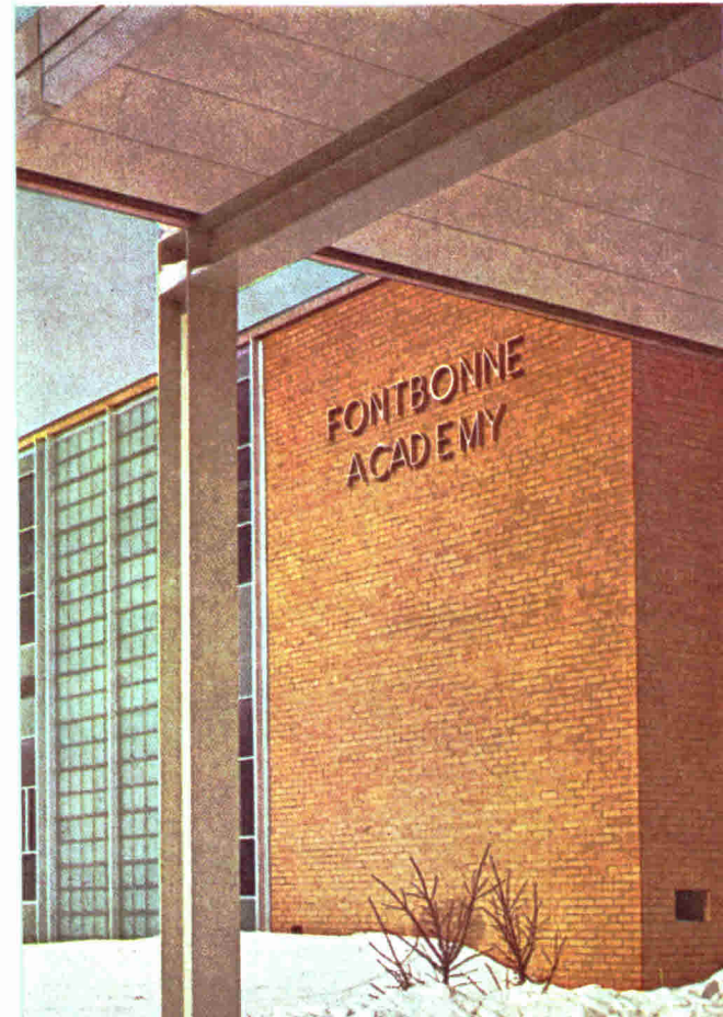
At Fontbonne Academy, Allegheny County, Pa., architects Celli-Flynn, McKeesport, combined light-controlling panels of green Thinlite with window and metal panels to achieve this unusual effect in the classroom wing. ▼
