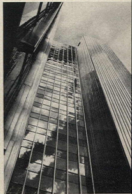
From any angle, Nickel Stainless mullions and external service tower give this new 22-story building top-to-bottom beauty. Interesting design note: colored Nickel Stainless strips are used on the service tower for strong vertical emphasis.
