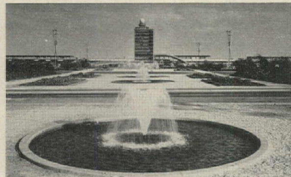
A thing of beauty is an underground pumping system
