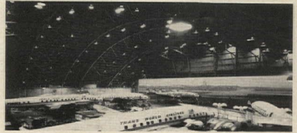
Interior of steel arch hangar, 300 by 218 ft, style 1 on page opposite, a PNYA design completed in 1950
