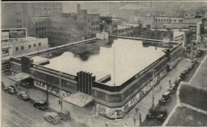
This 27 year old store of the J. C. Penney Company in Milwaukee has been given a million-dollar-plus remodeling job which involved everything but the water-cooled roof. Although the Koppers coal-tar pitch roof has been constantly under water for 27 summers, it is still in excellent condition, and should last many more years.
