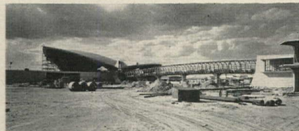
Transparent tunnel for passengers is also pressurized fresh air supply for satellite to keep jet fumes out
