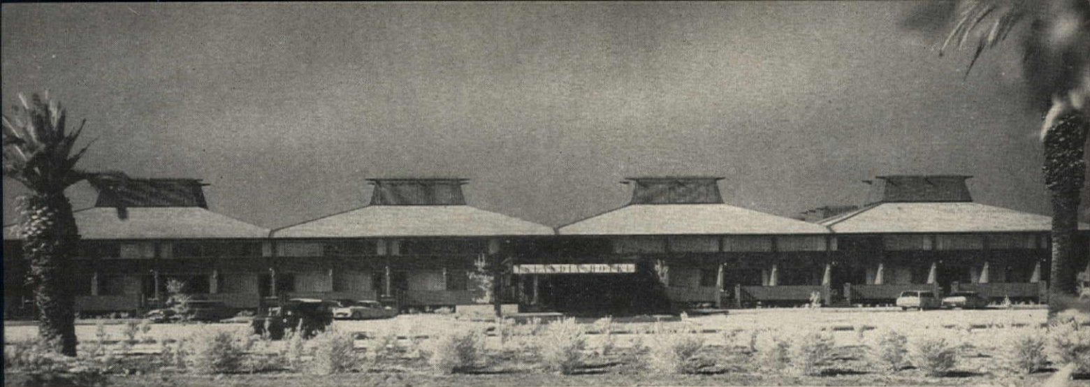
Slatted cupolas open second floor corridors to the sky and have great style
