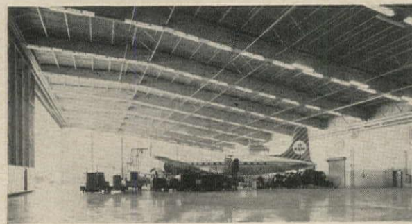
Hangar 17 has cable-supported cantilevered steel beams (above), a variant of style 6, a PNYA design
