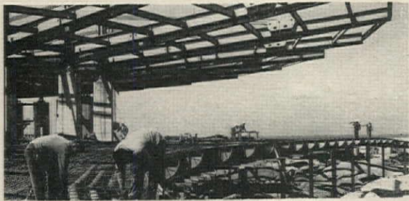
Framing for cantilevered canopy over PAA car ramp
