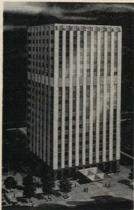
(far left) To be built under New York City's newly adopted zoning code, this $36 million 32-story office building designed by Skidmore, Owings & Merrill will occupy little over half the site. Structure will have masonry facade with horizontal sunshades. For two major tenants it will be divided in half functionally, with separate entrances, lobbies, elevator banks. Owner: Erwin S. Wolfson; contractor: Diesel Construction Co.
