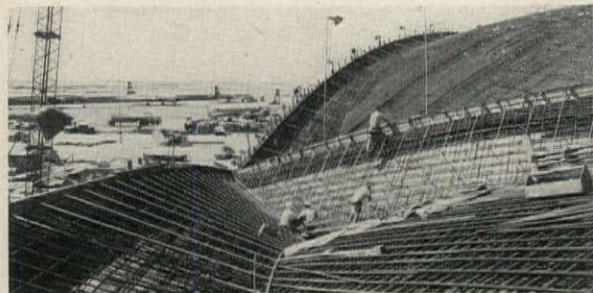
Laying steel on forms for a poured shell at TWA
