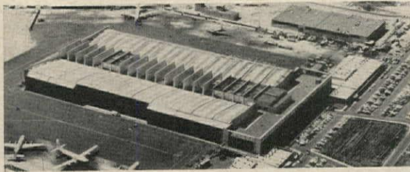
Air view of Hangar 14 shows how fin-like anchor walls for cables provide space for cooling towers and boiler
