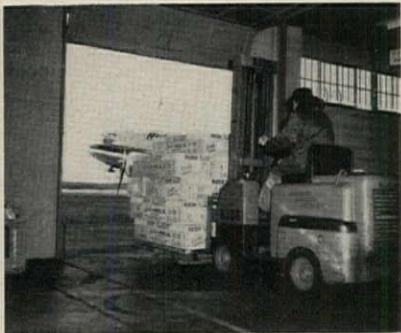
Clearances in one-story cargo buildings with 12.5-ft ceilings, 8 by 10-ft doors are designed for lift trucks
