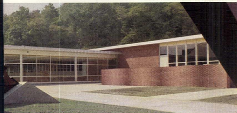
Beaver Area Senior High School, Beaver, Pa. Architect—B. J. McCandless, Ellwood City, Pa.
