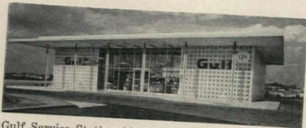
Gulf Service Station (Architect: Edward D. Stone)—complete automobile service in a building designed to complement Idlewild terminals and master plan
