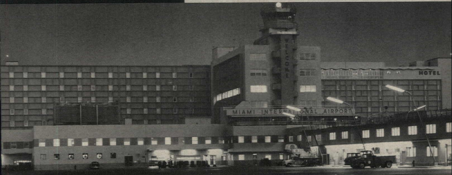
Miami International Airport, Dade County, Florida, one of the busiest airports in the United States and a world leader in air cargo. Building above is protected from loss of utility power with a dependable Cat Diesel Electric Set.
