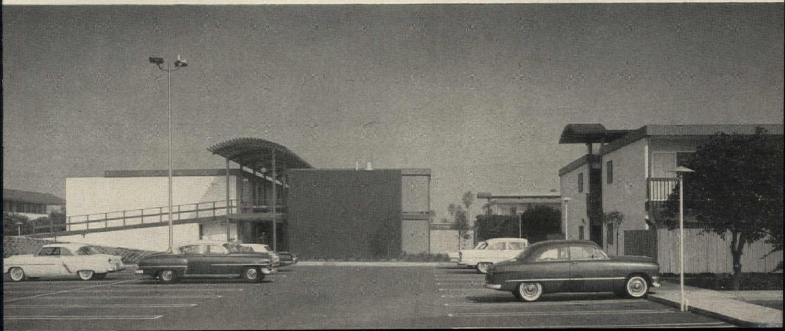
Blind walls abut parking. Ramps link guest room corridors to parking and are used by electric baggage carts
