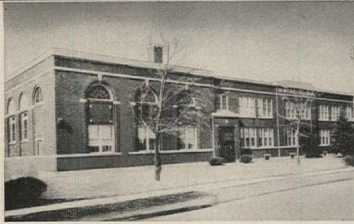
The original 20 year bond on the John A. Nichols School in Syracuse expired more than 12 years ago, but this Koppers roof continues to give trouble-free service year after year. Its coal-tar base is totally resistant to water penetration. No other built-up roofing material can offer 32 year service records like these.
