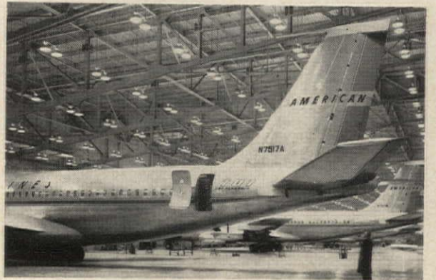
Cantilevered trusses soar over 43-ft tail of Boeing 707 in American Airlines' Hangar 10, a Kahn and Jacobs design in style 4, opposite, completed in 1958
