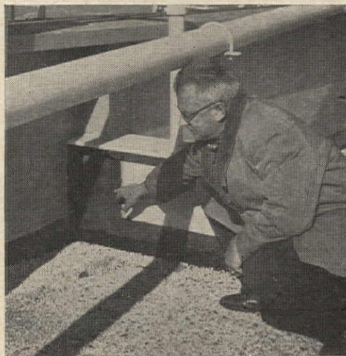
Saraloy accomplishes difficult flashing of bolted girder-purlin intersection
