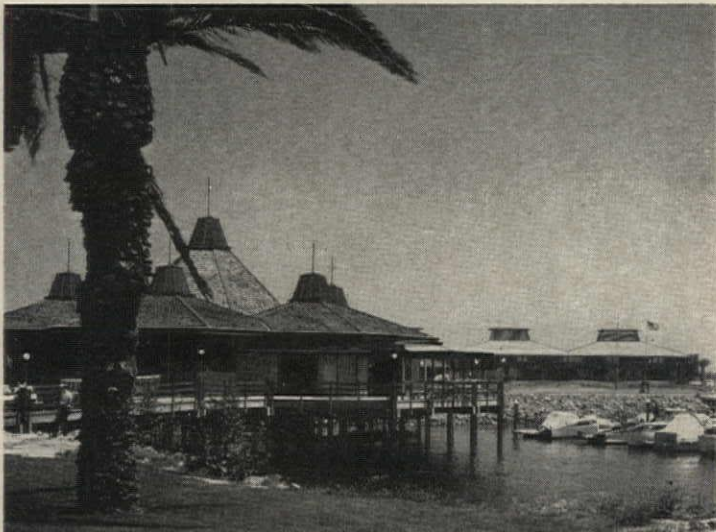
Restaurant is raised 15 ft above water on concrete piers
