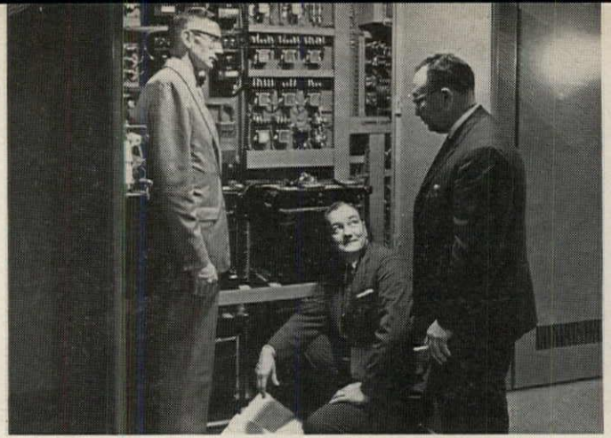
O. M. Newman, Heyl & Patterson, and Edward Cohen, Ammann & Whitney, discuss roof electrical drive with C. G. Falkenstein, Westinghouse, kneeling in front of main roof reactor control cabinet.
