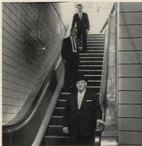
Type M Electric Stairway transports 8,000 persons/hr. Top to bottom: E. R. Gallagher, supervising architect; H. R. Helvenston, resident engineer; and A. Simmonds, Westinghouse Elevator.
