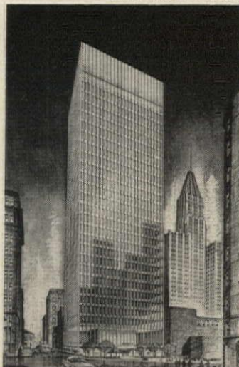
(right) Vincent Kling designed this 28-story square office building for Baltimore. To be completed by fall 1962, the 360-ft-high structure comprises approximately 400,000 sq ft. Exterior metal and glass wall provides deeply splayed window jambs for built-in sun control. Developers: Blaustein and McCloskey & Co.
