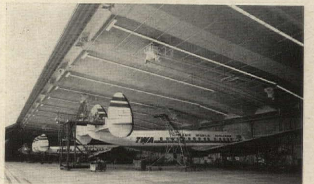
Amman & Whitney's prestressed folded plate, style 5, gives 50-ft clearance at TWA's Hangar 12, has less heated space overhead; note cable ties at beam ends
