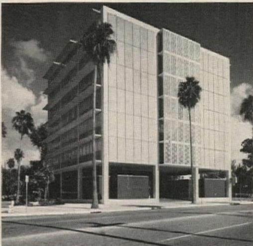
Ceco Adjustable Steelforms were used to create rigid concrete joist slabs in the Davis Building, Tampa, Florida.
