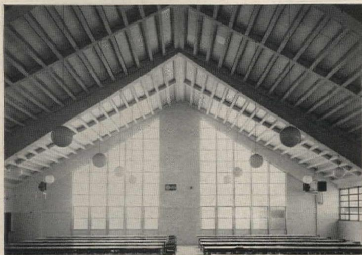
Special use of Ceco Longform Service resulted in this "beamed" ceiling in Jacksonville, Florida, Junior High School. Reynolds, Smith & Hill, architects and engineers Parker Construction Co., contractor
