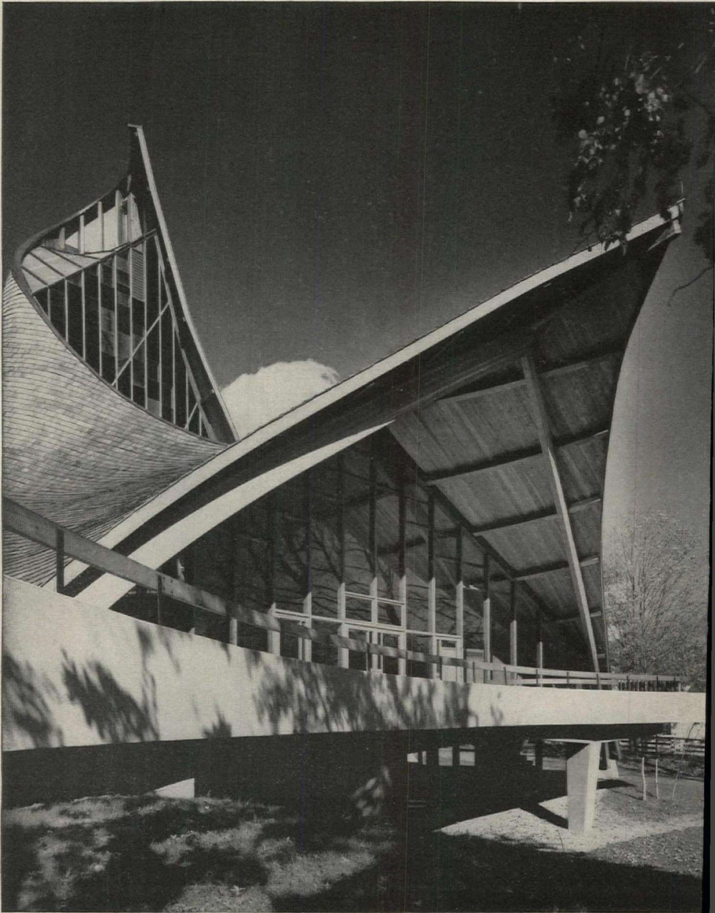
The heavenward spiral of wood shingles, laminated beams, and multi-toned planking makes the roof of the United Church in Rowayton, Connecticut, something spectacular. It demonstrates, too, the breath-taking wonders of wood's structural strength.
