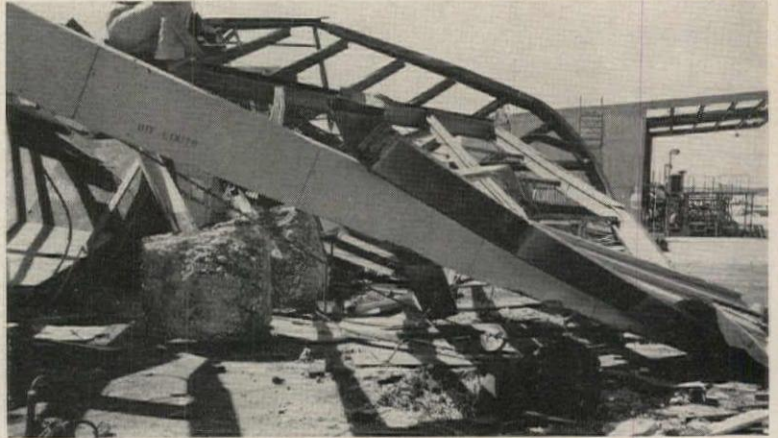
This light gage steel building was racked due to insufficient lateral bracing. Wind uprooted concrete footings of a nose hangar
