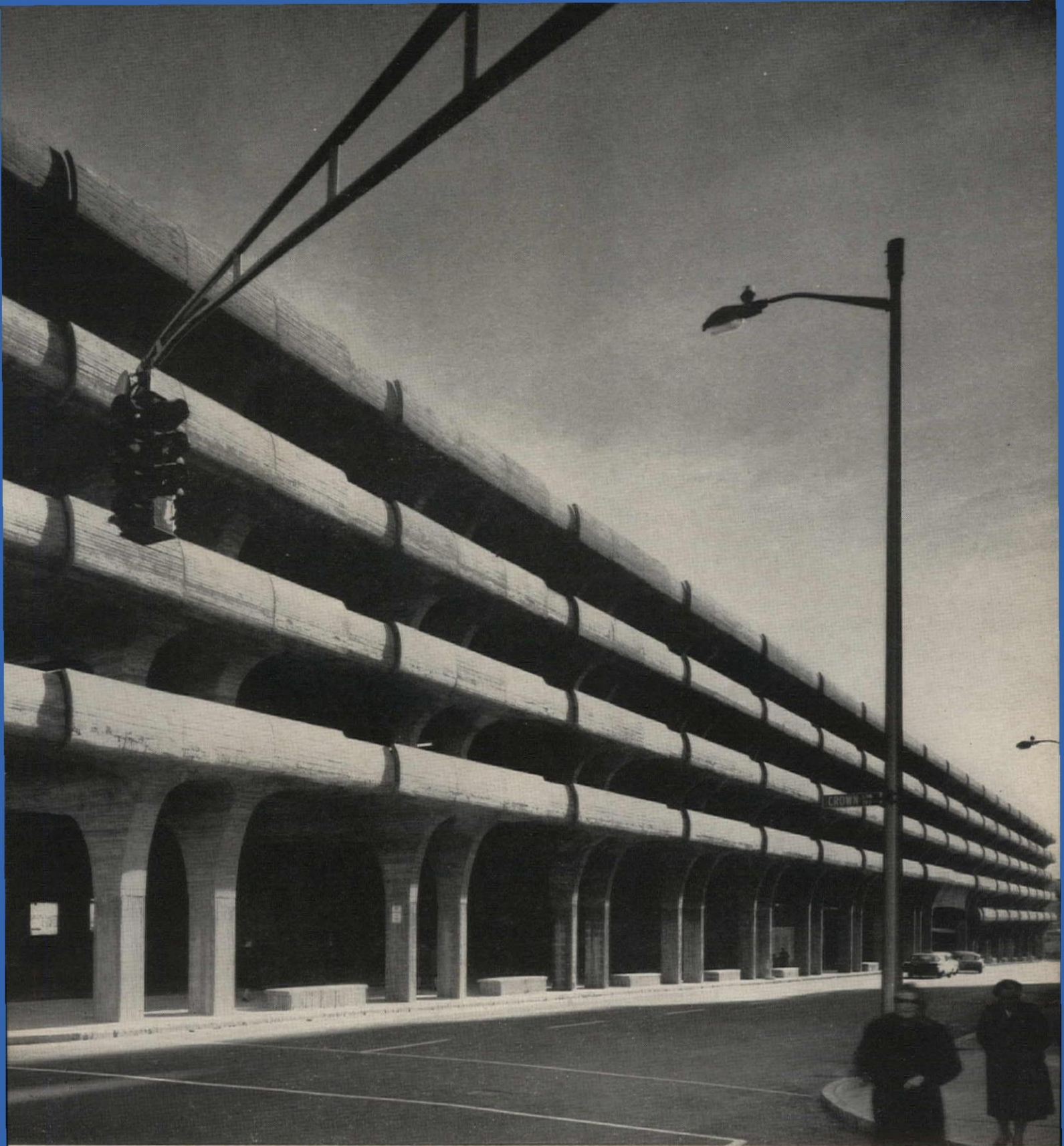
View from corner of Crown and Temple Streets near New Haven Green. The building is 118 feet wide and 726 feet long spanning a street to stretch across two city blocks to the edge of the Oak Street Connector which joins the Connecticut Turnpike. There is direct access to one of the garage's entrance and exit ramps from the connector. The garage will add 1,500 parking spaces to the 5,200 already available in downtown New Haven
