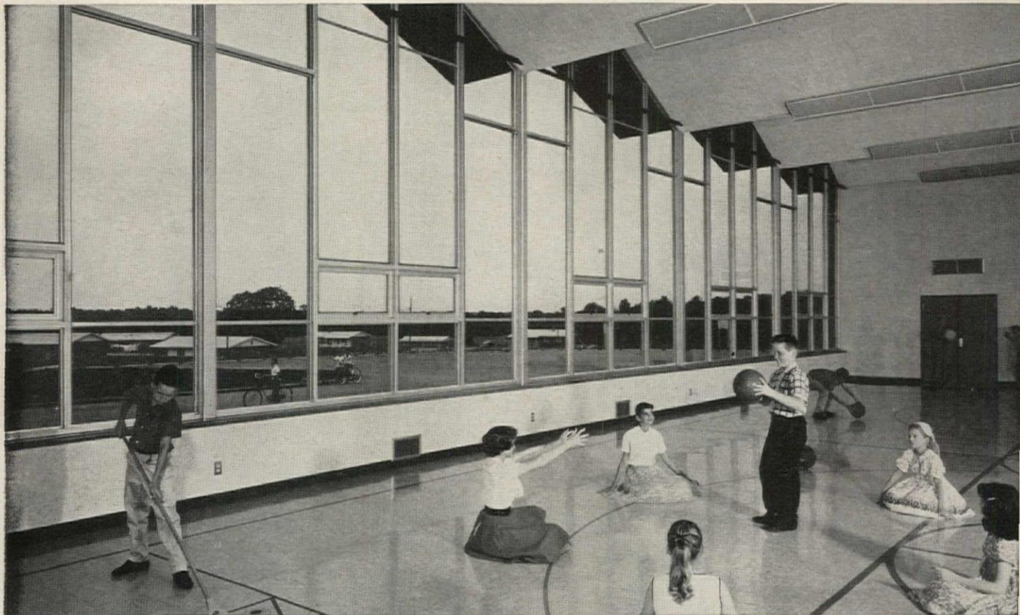
Window wall in gymnasium is glazed with Parallel-O-Grey Plate Glass that has been heat tempered for extra strength. Orchard Hills Elementary School, Novi, Mich. Architects: Charles W. Lane & Assoc., Ann Arbor.
