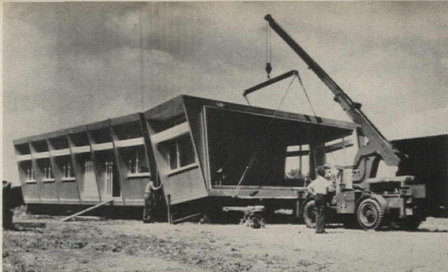
Portable school in Switzerland is assembled from easily transported sections; facade is slanted for sun control. Architects: Stuy and Meuli of Zug, Switzerland
