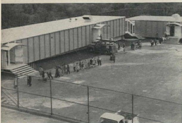
Floor, wall and roof panels and framing were assembled conventionally, but the school comes apart in 8-ft sections
