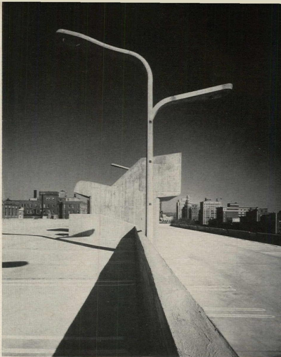
Rudolph insisted that concrete be used wherever possible even for such fittings as handrails and lamposts which would normally be of metal. Beyond the lamposts, which New Haven citizens call the twin cobras, is one of the penthouses which contains the elevator machinery and a great air intake fan
