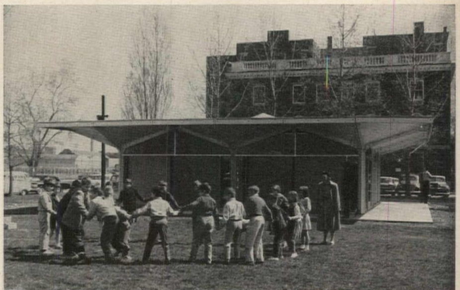
Demonstration model of M.I.T. classroom has exterior walls of glass and aluminum, plastic-core sandwich panels. One of the walls has built-in storage and encloses a self-contained heat pump
