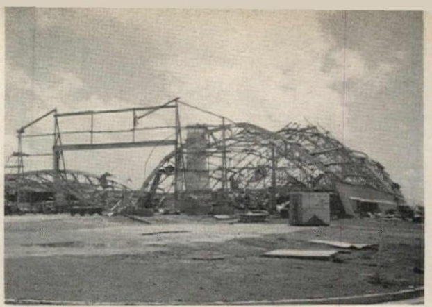
Loosely-anchored coverings were torn off. Debris damaged windows in housing. Lightly-framed arched hangar was destroyed
