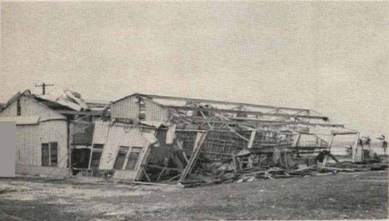
This light gage steel building was racked due to insufficient lateral bracing. Wind uprooted concrete footings of a nose hangar
