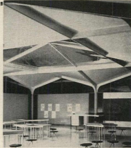
Top: Prototype classroom under construction. Flared column takes roof panels. Bottom: Model photographs illustrate potential interior and exterior designs
