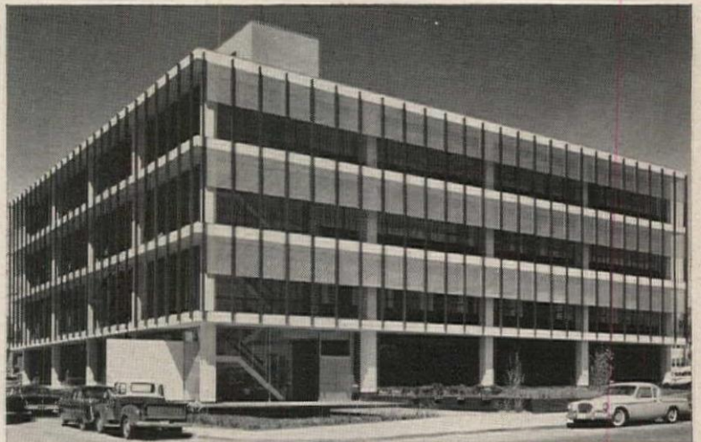
Office building for Old Security Life Insurance Company, Kansas City, Missouri, constructed with Ceco Flangeforms.
