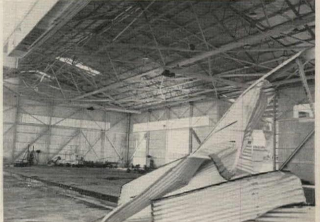
Wind blew off siding and glazing of hangar. Wind also apparently caused uplift on roof; then unanchored hangar door fell out
