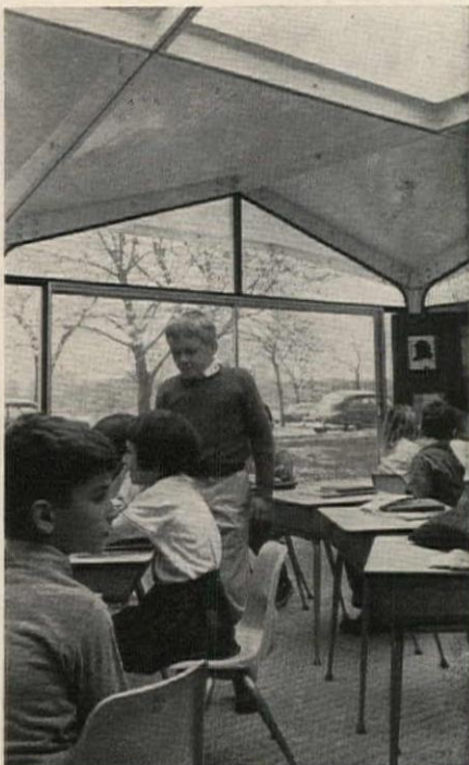
Demonstration model of M.I.T. classroom has exterior walls of glass and aluminum, plastic-core sandwich panels. One of the walls has built-in storage and encloses a self-contained heat pump
