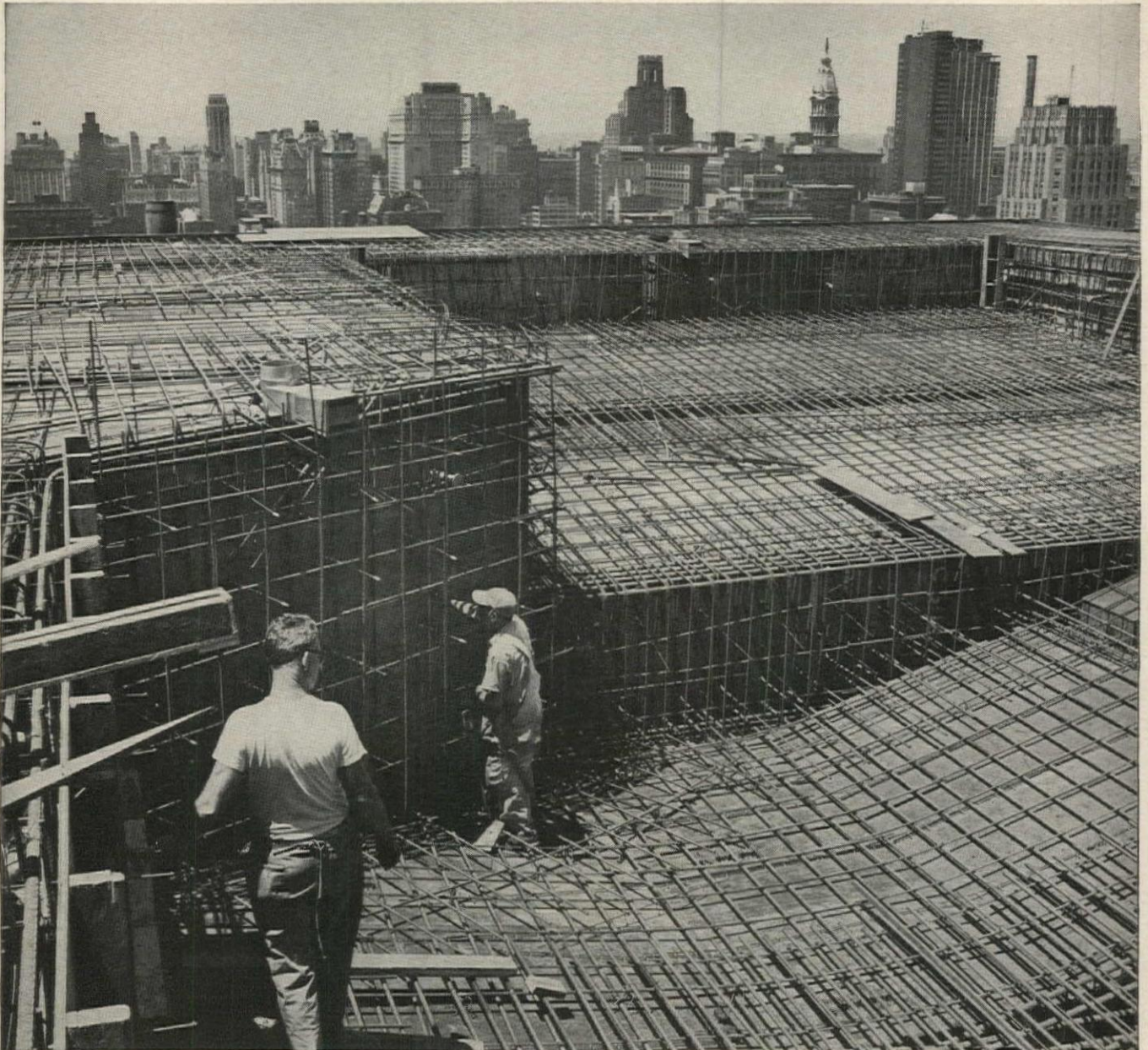
Bethlehem supplied 2,400 tons of steel reinforcing bars for the Hopkinson House Apartments in Philadelphia, including about 35 tons used in the rooftop swimming pool. Architect of the 35-story building: Stonorov & Haws, Garfinkel & Marenberg. General contractor: R. N. Shoemaker Co.; concrete contractor: Robert G. Hoffer Company; steel fabricator: Bethlehem Steel Company.
