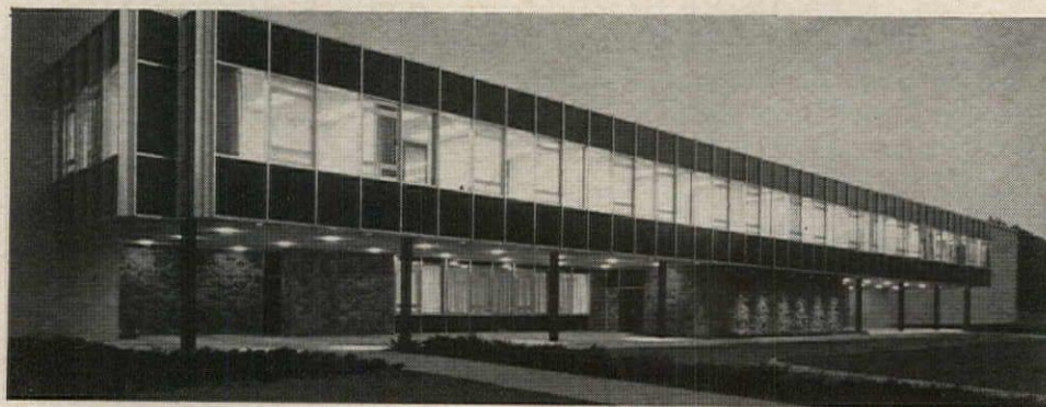
Alderman Studios' new 3-acre plant in High Point, North Carolina.
