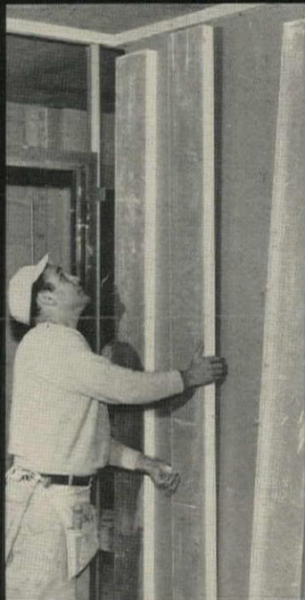
2. Apply adhesive-coated gypsum studs
