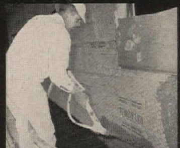
Cement trowelled prior to application of finish coat.
