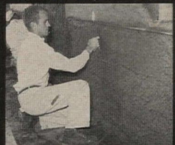
Cement trowelled prior to application of finish coat.
