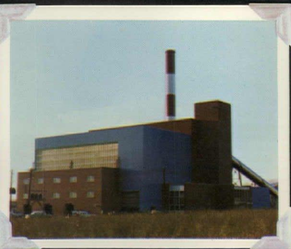
McKee Run Generating Station, City of Dover, Delaware. General Contractor; Somers Construction Co., Bala Cynwyd, Pa.
