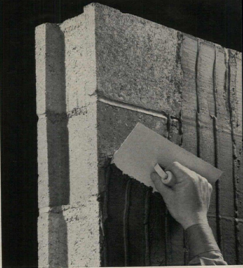
2. Start with Styrotac® bonding adhesive.
