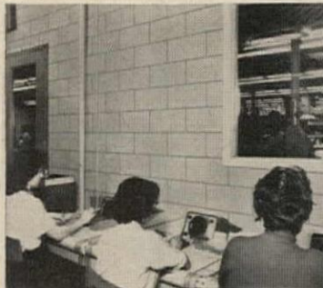
The block of Natco Vitritile shown on right is the 8-W series in the nominal face size of 8" x 16". The production area on the left shows typical installation.
