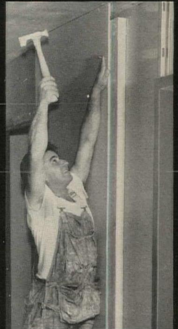
4. Apply back face layer to runners and studs
