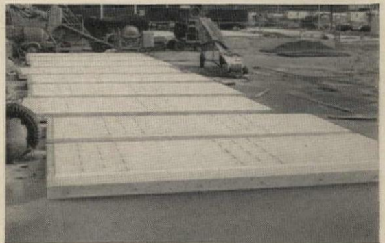
Reinforced concrete slabs—each 8 feet 4 inches high, 20 feet wide and 8 inches thick—are used for walls of manufacturing and warehouse sections. Slabs are laid horizontally tongue-and-groove fashion to form wall sections 25 feet high by 20 feet wide.
