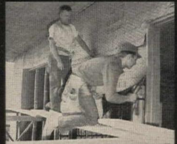
Portland Cement is sprayed on.
