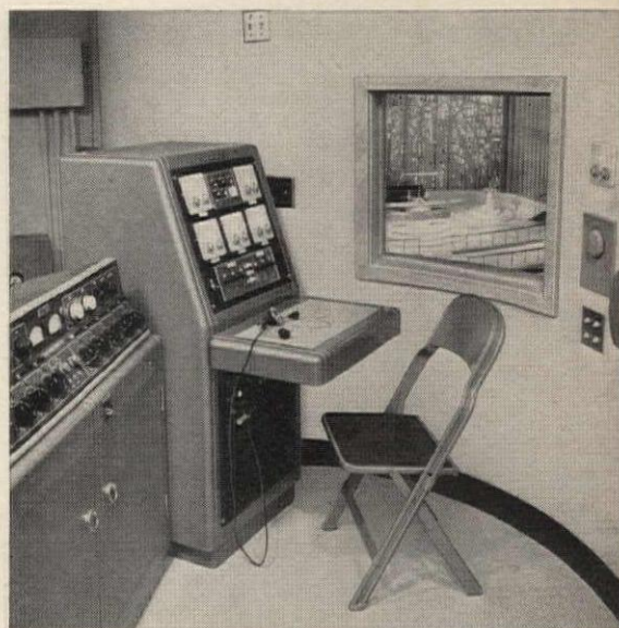
While the entire system may be controlled from this control room overlooking the sanctuary, other switches are placed throughout the church for the convenience of the minister, ushers, the organist, and the sound technician.
