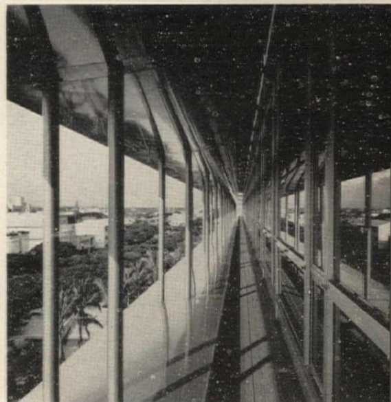
Neoprene gaskets between 10-ft lengths of sun-blades allow thermal expansion
