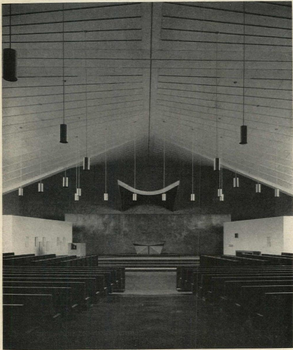
The main chapel can be seen in the two photos ( above ). The exterior buttresses of rough concrete take the lateral thrust of the chapel roof, composed of four half-hyperbolic-paraboloid shells. The high edges of these shells conjoin along a central axis, leaving the interior space free of supports. The concrete roof and fieldstone walls are painted white inside; the reredos screen is gold leafed; the baldachino is lacquered primary blue; the floor is polished black brick; the pews are of dark-stained oak
