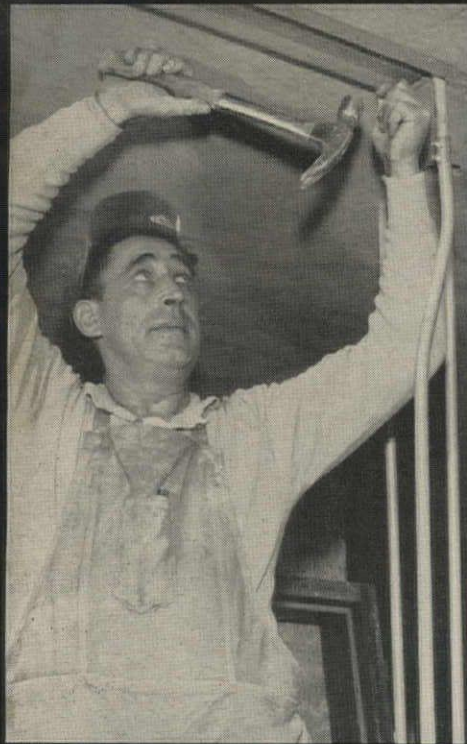
A. Install metal floor and ceiling runners
