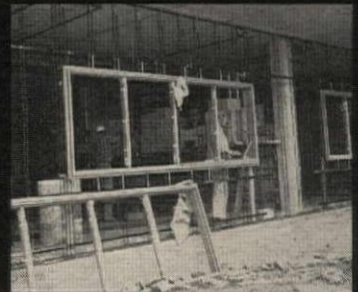
Then Keymesh Paperbacked lath is applied.
