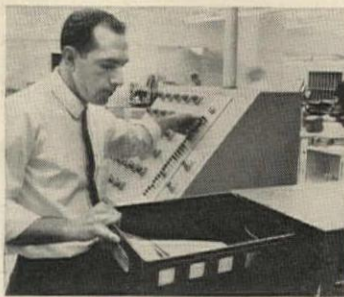
Mail room clerk sends basket to designated floor simply by pushing a button. Each tote box carries up to 32 lbs. of payload... the conveyor accepts up to 12 loads a minute.
