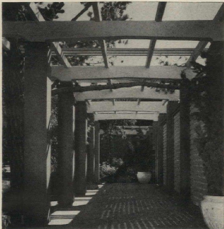
Latticed walls, square columns, and arched and criss-crossing members of wood overhead form a sunny welcome for a walkway entrance to this contemporary home; show still more of wood's wealth of uses.
