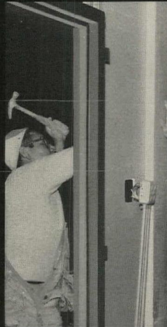
3. Secure gypsum studs with nails or screws
