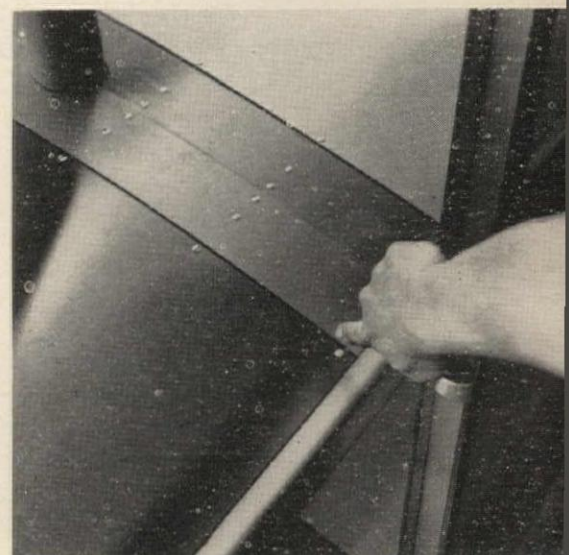
Neoprene gaskets between 10-ft lengths of sun-blades allow thermal expansion
