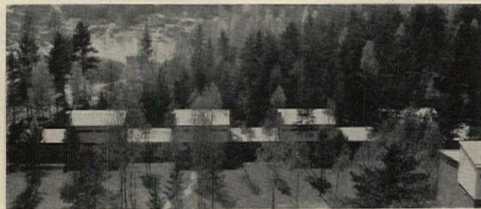
Terrace houses; Aulis Blomstedt, architect
