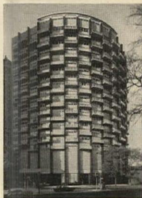
Windsor Apts., Philadelphia, Pa.; Architect: Aaron Colish; Painting Contractor: M. Schnoll & Sons; Man from Devoe: George Mac- Naughton—all of Philadelphia.
