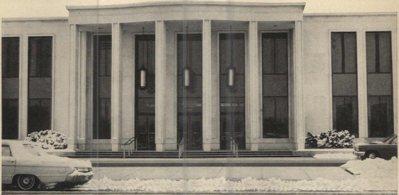
New $3,500,000 Associates Investment Co. home office has SNO-MELTER Electric Heat Mats beneath customer walks, driveways, shipping docks. Only the results show!
