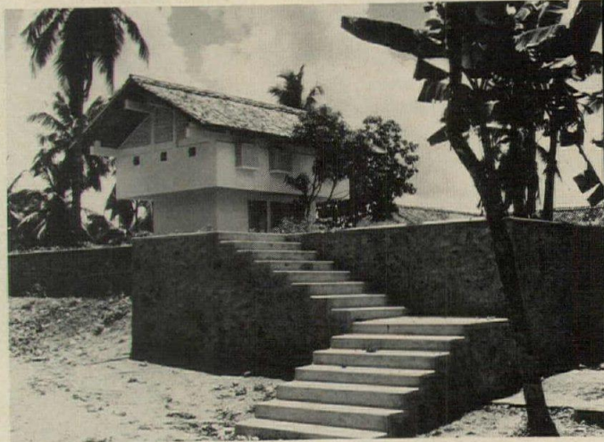
Pan Pacific Citation from Hawaii Chapter, A.I.A., and The State Foundation on Culture and the Arts: to architect Geoffrey Bawa, a partner in the firm of Edward, Reid and Beggs of Colombo, Ceylon, for "excellence in design." Shown here is the Infirmary at the Good Shepherd Girl's Town, Hannella, and on page 5, at bottom, the smokehouse and curing facilities at Girl's Town.
