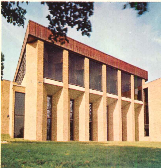
The functional and highly decorative band which terminates Agudath Sholom Synagogue (left and above) in Stamford, Conn., is an excellent example of a typical copper fascia. Architects: Davis, Brody & Associates.
