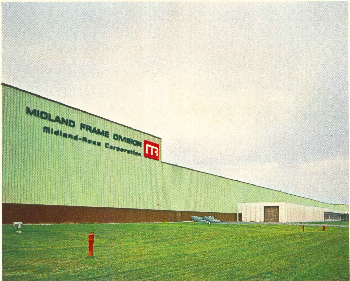
Frame Division Plant. Owner: Midland-Ross Corporation, Maumee, Ohio. Contractors: Lathrop Company, Toledo, Ohio. Engineers and Architects: Rossi & Nickerson, Toledo, Ohio. Finish: Metal walls finished with Fluropon† made with Kynar 500.
