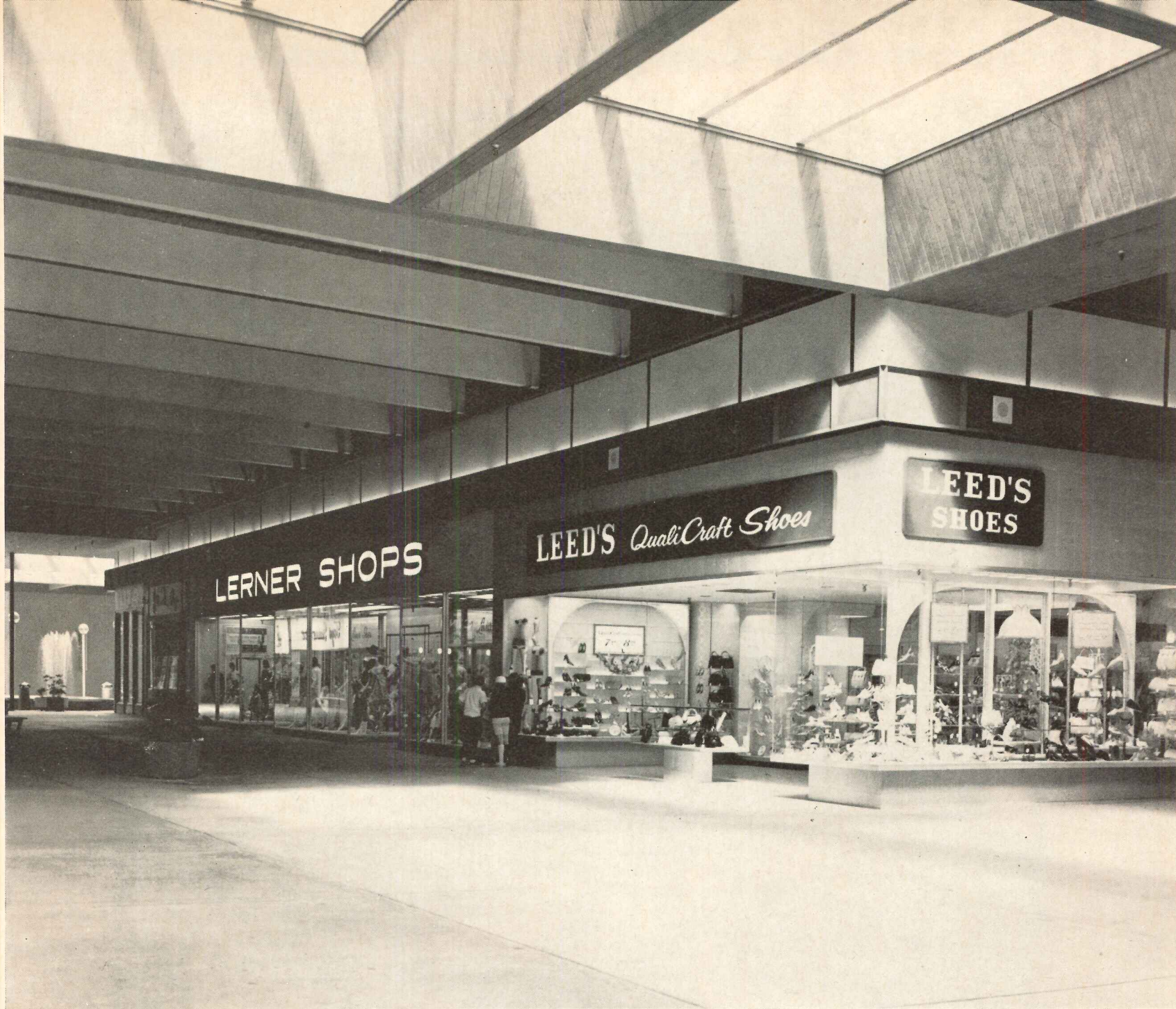
Lacey, Washington's modern South Sound Shopping Center is heated and cooled by Lennox rooftop heat pumps. Stores, bakeries, music shops, drugstores, restaurants and malls are among the areas with high-occupancy problems. Here the simple-to-install, single-package heat pumps provide the "micro-climates" required for the varied comfort control zones. Architect: Robert T. Olson, A.I.A. Engineer: Robert W. Platt.
