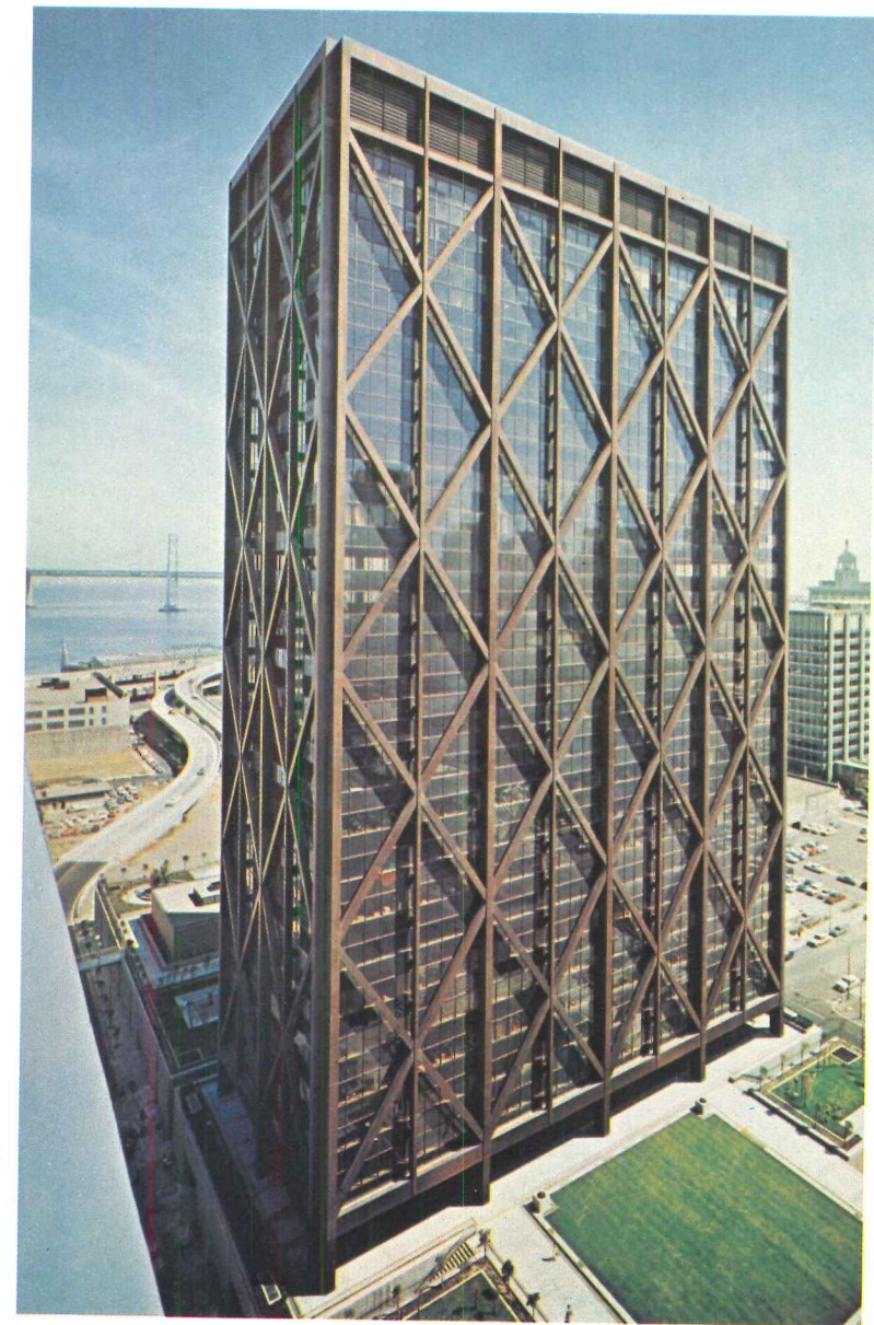
Alcoa Building, San Francisco, California "Here is a landmark structure which introduces a handsome bracing system to the San Francisco skyline. The structural system produces an interesting facade and provides stability against wind and earthquakes. It is ideal to this geographical location."
