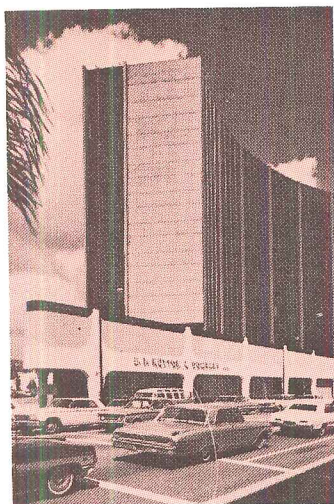
WILSHIRE TRIANGLE CENTER BEVERLY HILLS, CALIF. Architect: Sidney Eisenstat, AIA Curtain Wall Panels: Soule Steel Co. Sealant Contrs: Security Builders
