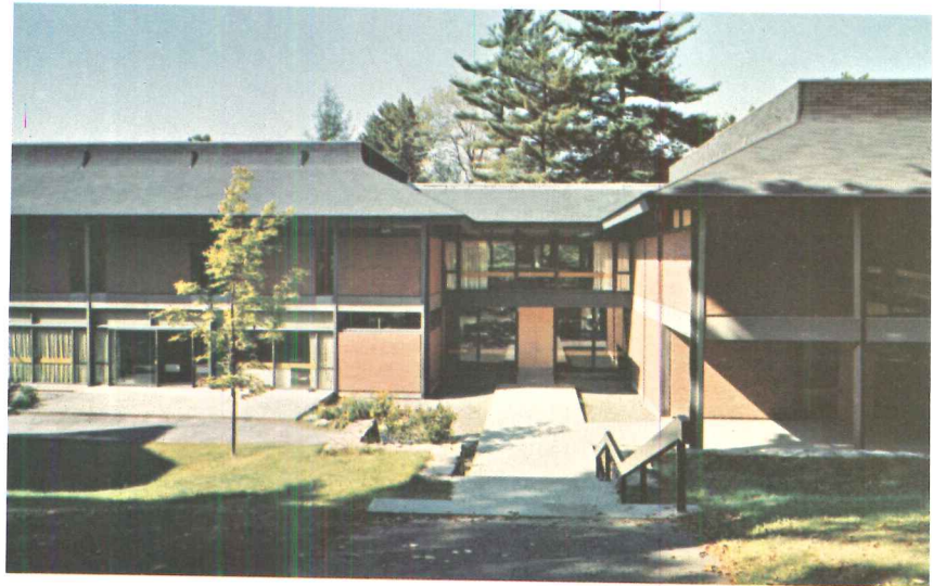
C. Thurston Chase Learning Center of Eaglebrook School, Deerfield, Massachusetts "Steel and masonry are used well together to create a warm environment for learning that maintains the human scale and avoids an institutional feeling."
