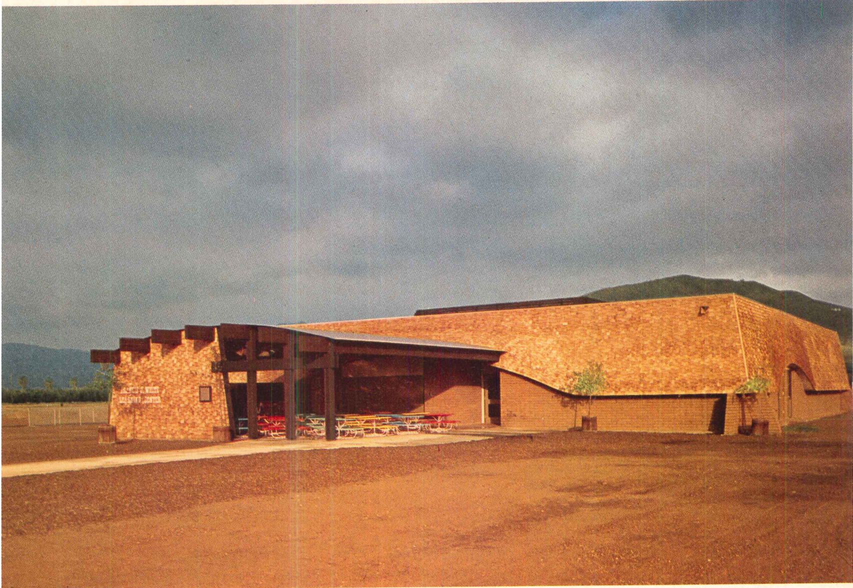
Francis J. White Learning Center, Woodlake, California. Architect/Engineer: Moring & Hayslett. Roof treatment completely conceals Lennox rooftop equipment.
