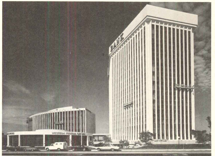
The Del Amo Financial Center, Torrance. Victor Gruen Associates. The project "contains the first modified ductile frame, reinforced concrete high-rise building designed to meet the new seismic code requirements of the City and County of Los Angeles."
