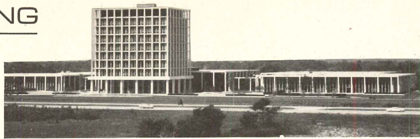
Ten stories of dramatic architecture and a complex of satellite buildings house the Allstate Insurance Companies in Northbrook, Illinois. Under roof are 722,783 square feet of functionally attractive work areas such as this computer center.
