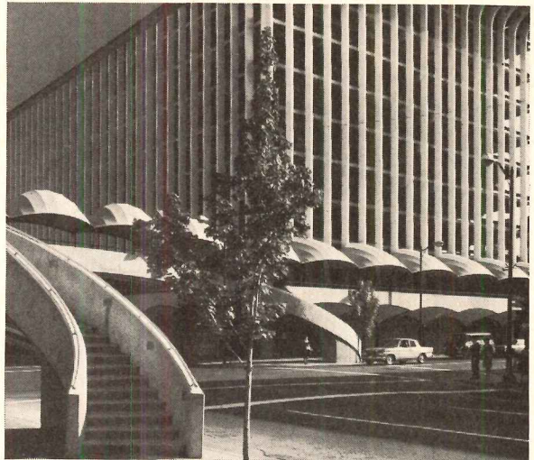
This beautiful facility provides off-the-street parking for 936 cars in the heart of downtown Spokane. Dimpled, textured precast fascia panels were used on the second floor of the structure as well as on the skywalk leading to an adjacent store.
