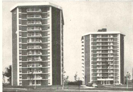
Stephen J. Collins Elderly Housing "Twin Towers" Architect: Caolo & Bieniek Associates Engineer: Greenleaf Associates
