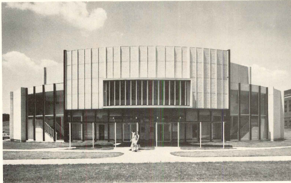
Theater and Classroom Building, Birmingham-Southern College, Birmingham, Ala. Architects: Warren, Knight & Davis. Theater Consultant: Dr. Arnold Powell. General Contractor: Brice Building Company, Inc. Dover Stage Lift installed by Dover Elevator Co., Birmingham.
