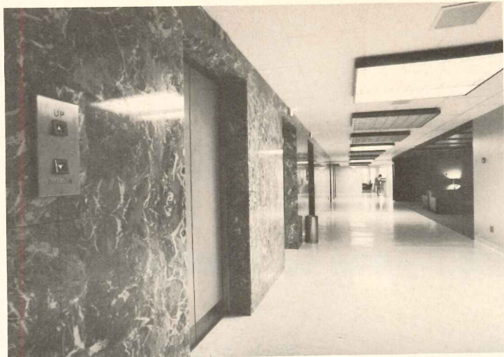
Typical floor area protected by emergency lighting circuits shows one passenger elevator operating; every third fluorescent fixture is lighted.
