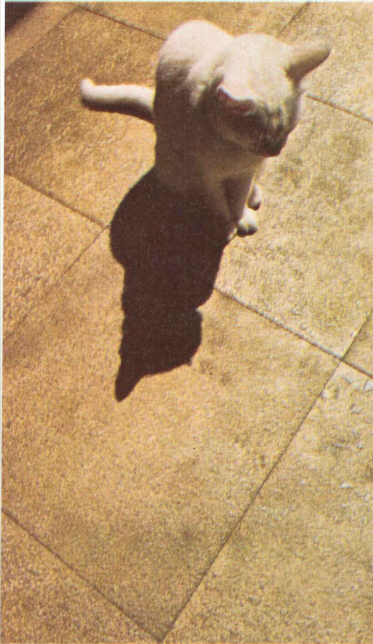
Bronze floor tiles (left). Pebble textured bronze on copper sheet applied directly to concrete or plywood. Needs only minimum care. Foot traffic adds varied highlights of muted gold tones.
