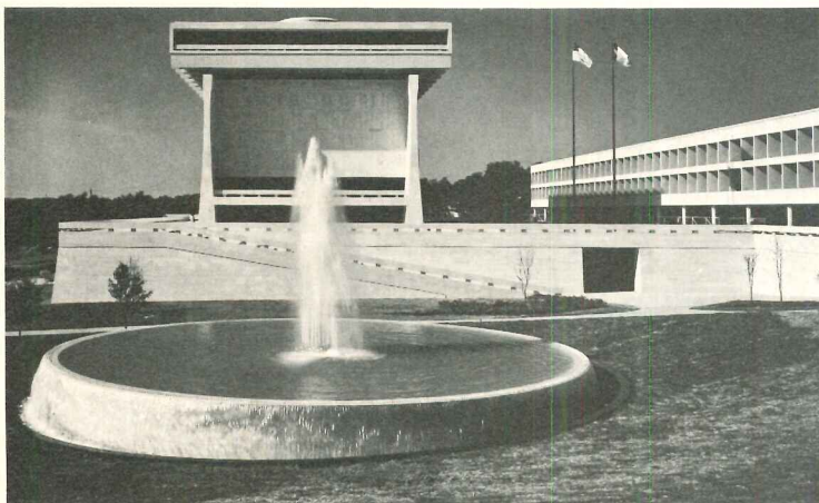
The Lyndon Baines Johnson Library , University of Texas, Austin, Skidmore, Owings & Merrill, Brooks, Barr, Graeber & White, architects, is becoming known as Lyndon's Pyramid. The combined museum and library is an eight-story monolithic structure with an 85 ft square and 55 ft high Great Hall with one glass wall exposing five levels of archives.
