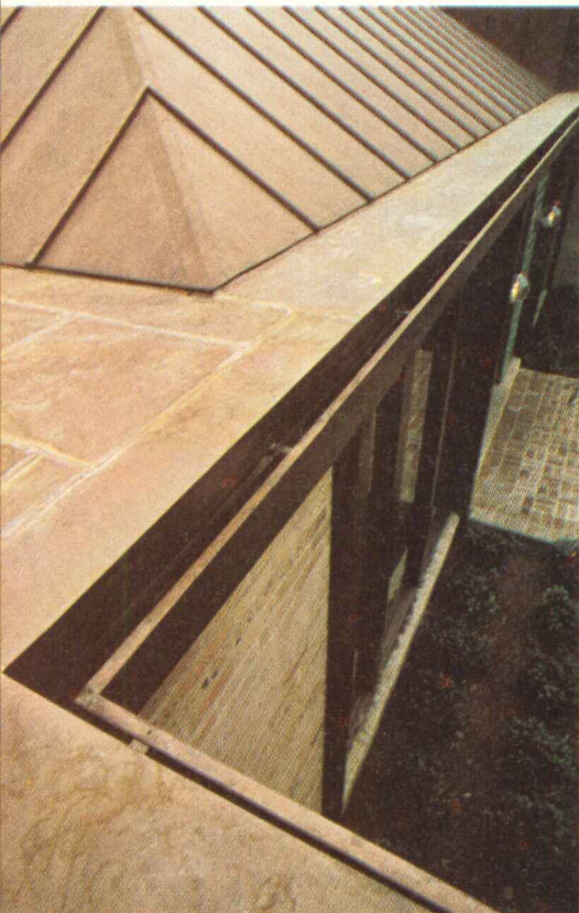
Copper gutters and flat roofing (above). Corrosion-resistant copper is as functional as it is beautiful. Highlights quality.
