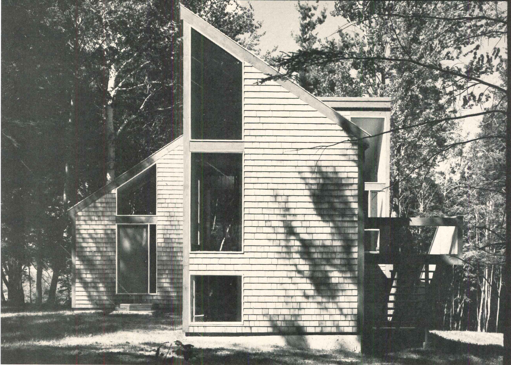
Vacation home at Francestown, New Hampshire. Certigrade Shingles No. 1 Grade 16" Fivex. Architect: Brett Donham.
