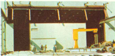
WITH POSTS OUT-OF-THE-WAY, THE OPENING IS COMPLETELY CLEARED — UNOBSTRUCTED.
