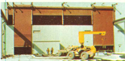
POWER OPERATED INTERMEDIATE POSTS AUTOMATICALLY RAISE AFTER DOORS OPEN.
