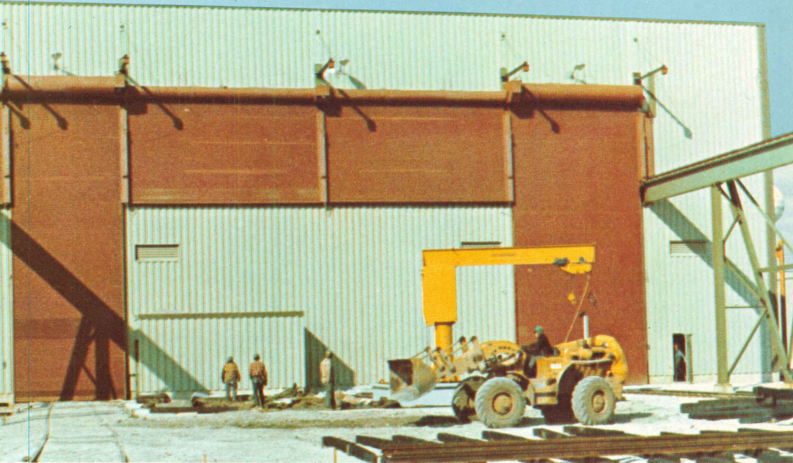
THIS LARGE CRANE OPENING IS COMPLETELY CLOSED WITH KINNEAR MOTOR OPERATED DOORS.
