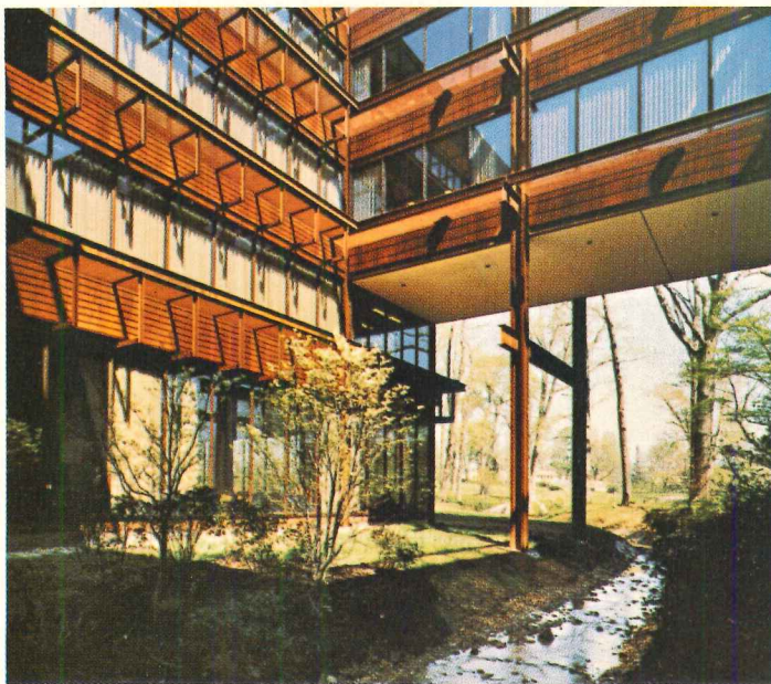
Weathering Steel gratings at each floor level, between the exterior walls and the sun screen, facilitate washing the bronze-tinted insulating glass.
