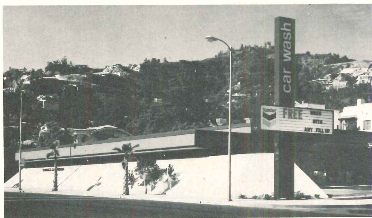
Sunset Car Wash on West Hollywood's Sunset Strip by Robert L. Barnett Associates has massive sloping poured concrete walls which shield the car wash machinery from view and shield the neighborhood from noise, water and suds. Its
