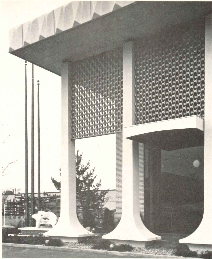
Manners Executive Office Building, Cleveland, Ohio Architect: Armet & Davis, Los Angeles, California. Contemporary C-20 Facade Screen, satin-gold finish. Seven panels, each measuring 100 square feet.
