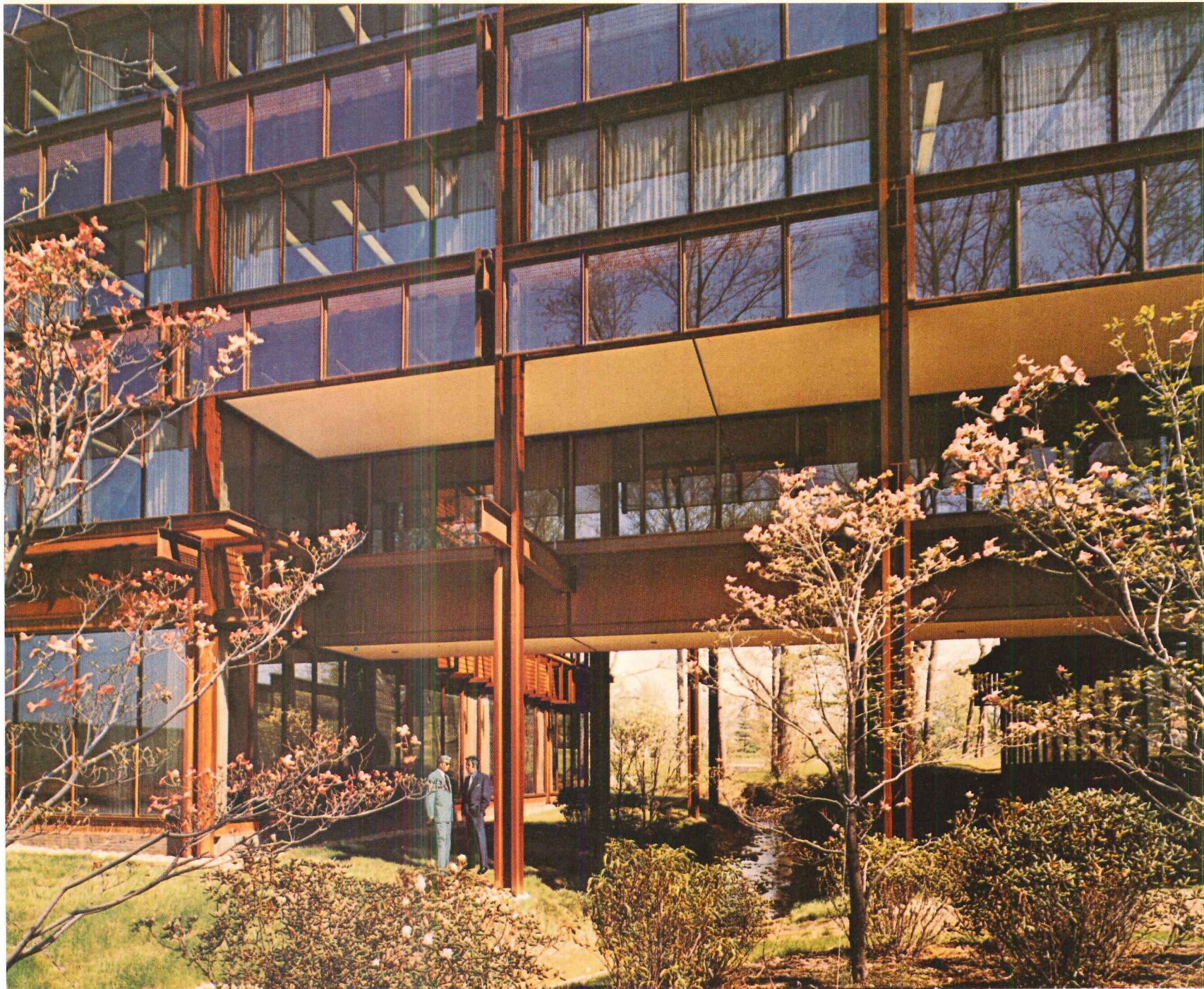
The central section of National Liberty Corporation's new headquarters bridges a valley and a small stream crossing the site. An artificial lake further enhances the landscaping while an existing adjacent wooded area is maintained intact.
