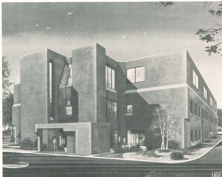
The Kirkwood/244 Medical Arts Facility in St. Louis by Martin Bloom Associates, Inc. is programmed to have pharmaceuticals and a laboratory on the first floor; the remaining floors are potential lease areas. Structurally the building combines exterior bearing masonry walls with internal steel frame.
