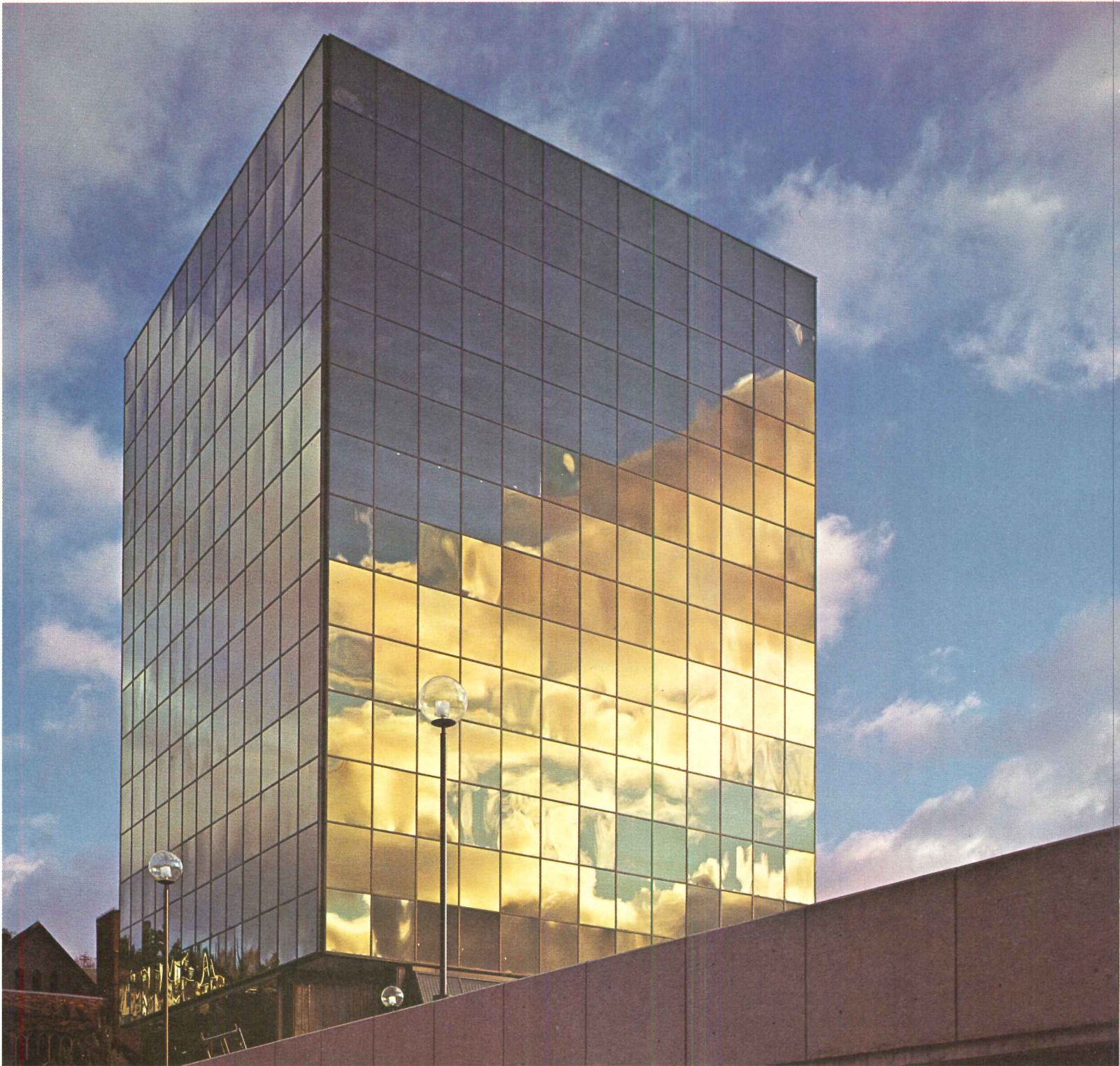
Owners: Detroit & Northern Savings & Loan Assoc.; Architect: Maurice B. Allen, Jr., A.I.A., Tarapata-MacMahon-Paulsen Corp., Bloomfield Hills, Michigan
