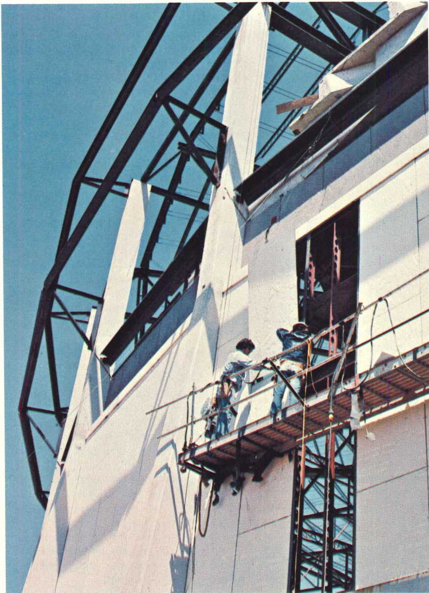
Exterior walls of the new Huntsville, Alabama, Civic Center are J-M Stonehenge® architectural panels secured directly to the steel studs. Here insulation is sprayed on the back of the panels. A combination of hidden and reveal joints was chosen by the architect.
