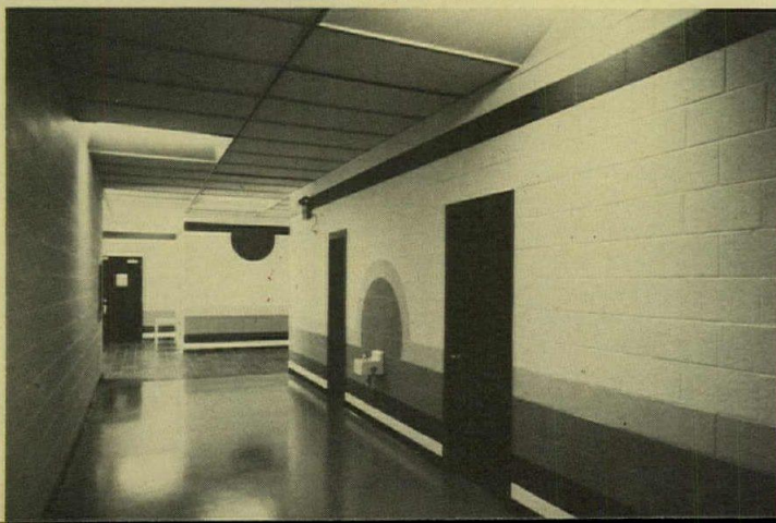
In a recent, abbreviated third phase, SEF had to forego some subsystems to cope with costs. Exteriors were split block instead of precast panels; electrical distribution and communications were conventional. Lighting was of similar good quality. Areas were cut down. Interiors were made cheerful by the choice of colors and tasteful designs in paint.
