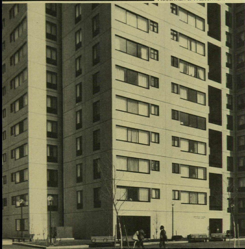
Precast concrete systems for high-rise housing have been imported from Europe , hopefully to make inroads into the still vast need for habitation. Some systems are in financial difficulty because of logistical problems, because of their plant amortization costs and because of a variety of management problems. Quality of product often has been excellent. This building for UDC is in Rochester's Southeast Loop. Architects: Hoberman & Wasserman.
