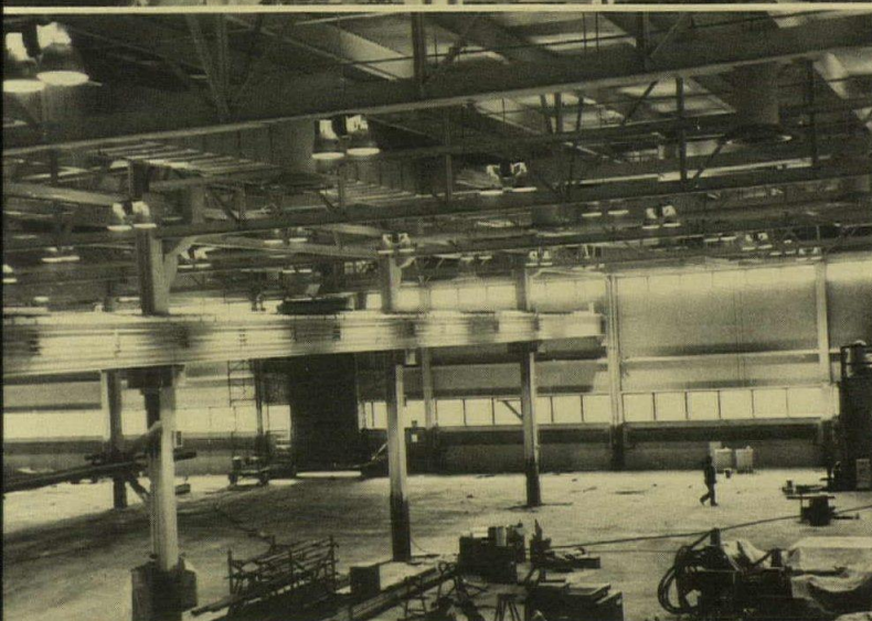
The crane runway beams are shown in the photo above. Below is a view of a mezzanine.
