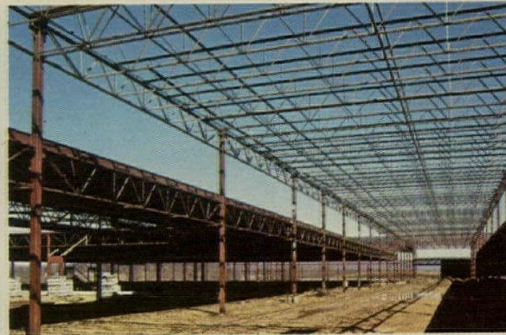
The high strength of steel joists and joist girders provides increased clear span area, allowing larger bays.
