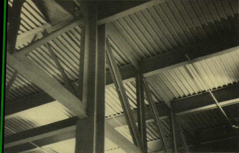
Roof trusses are shown at a column. The smaller diagonals are in the stiffening truss.
