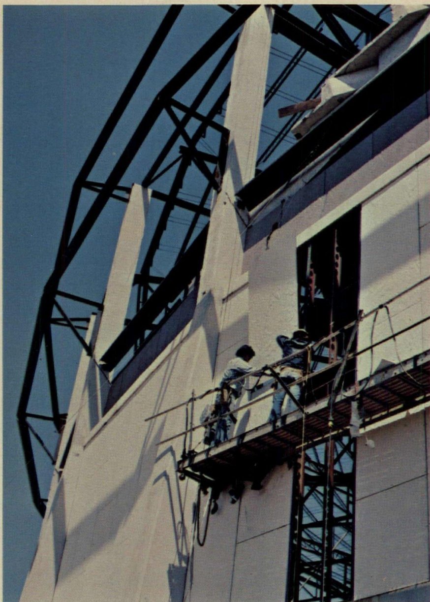
Exterior walls of the new Huntsville, Alabama, Civic Center are J-M Stonehenge architectural panels secured directly to the steel studs. Here insulation is sprayed on the back of the panels. A combination of hidden and reveal joints was chosen by the architect.
