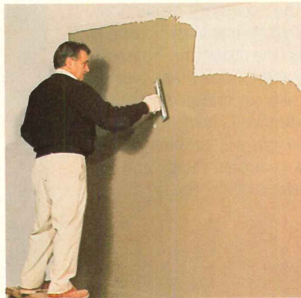
with its factory laminated fiberglass mesh, is applied to the gypsum board. In the second photo, the strong, cementitious prime coat is troweled over the insulation. And in the third photo, the
