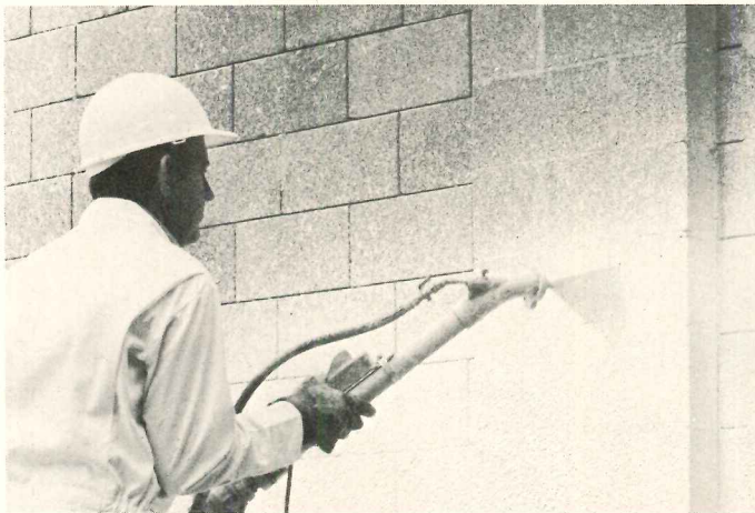
Spraying is the fastest way to apply BlocBond. Three men can cover about 1200 sq. ft. an hour.
