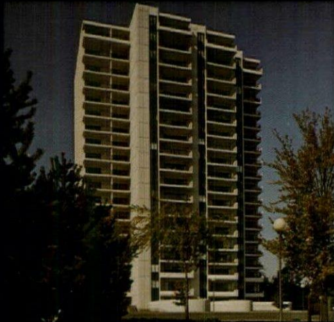
AMERICAN PLAZA TOWERS PORTLAND, OREGON
