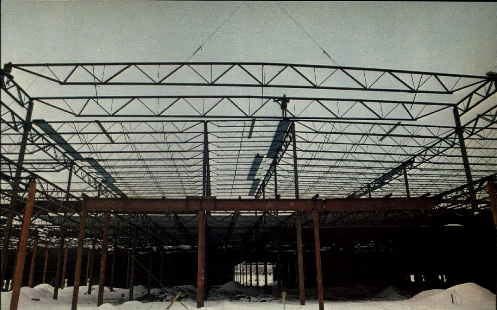
Use of 100' long span joists and 30' joist girders created a large clear span area in the center section of this enclosed shopping mall.
