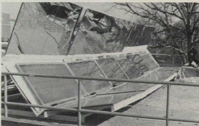
Roof structure of Shenandoah Community Center was designed to accommodate the solar-collector array. Web members of the wood roof trusses are at the angles chosen for maximum system efficiency—45 degrees on south slopes for the collectors and 36 degrees on north slopes for the polished aluminum reflectors. All walls have earthen berms except the north which is 40 per cent insulating glass.
