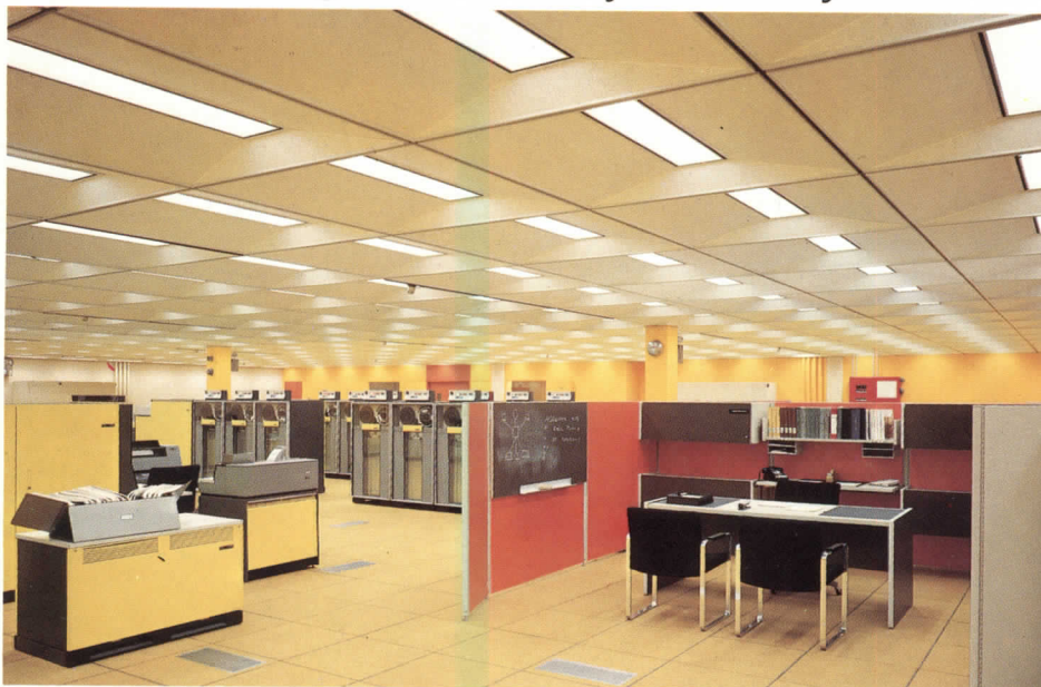
Datacenter/The Equitable Life Assurance Society of the United States, Easton, Pennsylvania, Architects: Kahn and Jacobs, New York City, Ceiling System: Armstrong C-60/60 Luminaire
