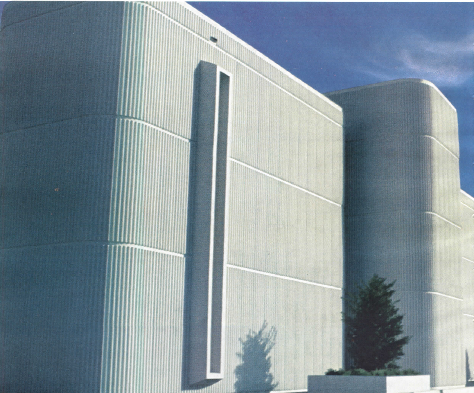
Louis Calder Memorial Library, Miami, Fla. • Arch.: Steward & Skinner Ass. • Contr.: Clark Construction Co. • Appli.: Bernard Snetiker Painting Contr.
