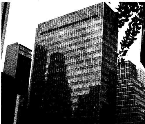
Lever House New York, New York, sealed with Thiokol polysulfide base sealant, 1954
