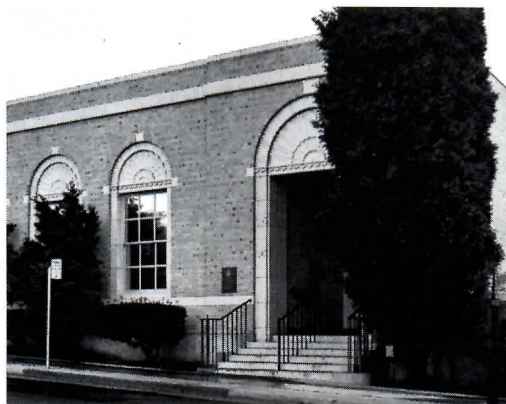
California Telephone & Telegraph Building Albany, New York, sealed with Thiokol polysulfide base sealant, 1947
