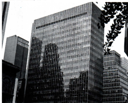
Lever House New York, New York, sealed with Thiokol polysulfide base sealant, 1954
