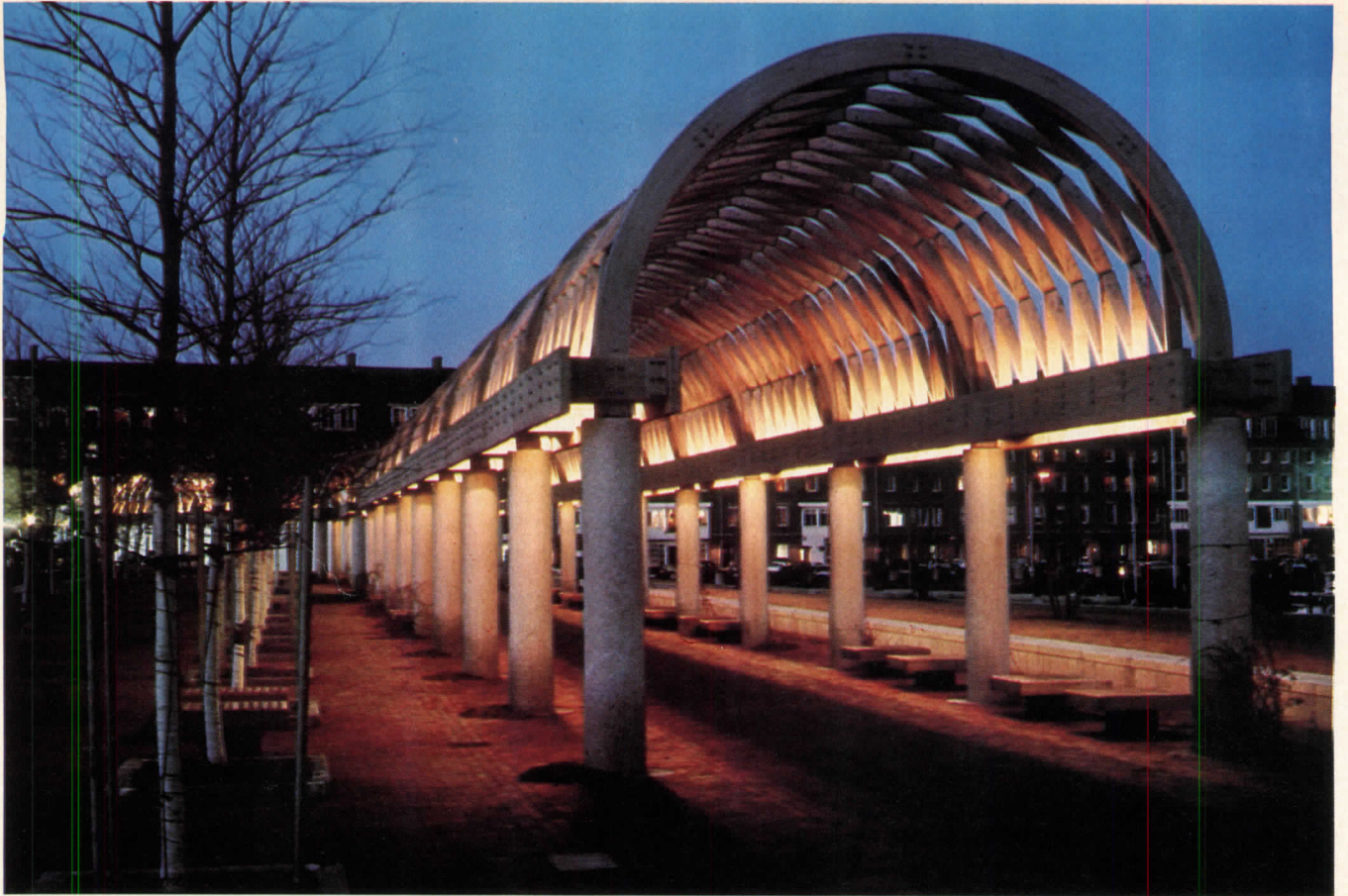
Laminated wood trellis at Boston Waterfront Park, Boston, Mass. Wood structure supplied and assembled by Unadilla Laminated Products, Unadilla, N.Y. Architect, civil engineer, landscape architect: Sasaki Associates, Inc., Watertown, Mass.
