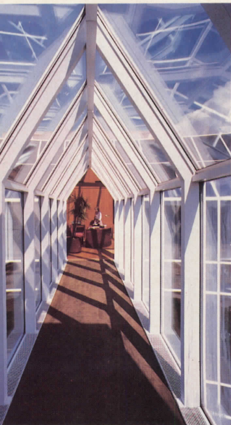
A steel-framed pedestrian bridge (above) connects the free-standing elevator tower to the garage, ground, and third levels. The concave facade (left) emphasizes the entrance and preserves as much of the landscape as possible.
