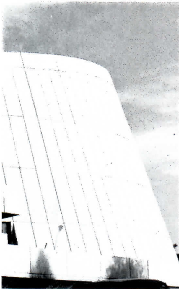
The visual effect of form butt-splice joints appears in the spandrel beam of the top photo (shown more completely on the opening page). Plastic-coated plywood and revealed joints give still a different treatment for a wall in the Indiana University Museum of Fine Arts (center, right) Architects: I. M. Pei & Partners; engineers: Weidlinger Associates. The truncated cone over the auditorium of Herbert Lehman High School in New York City (above) has revealed joints. Vertical reveals are approximately 4 ft apart at the base. Control or construction joints were introduced at the reveals every 12 ft; Architects: The Eggers Group P.C.; engineer: Frank Burgess.
