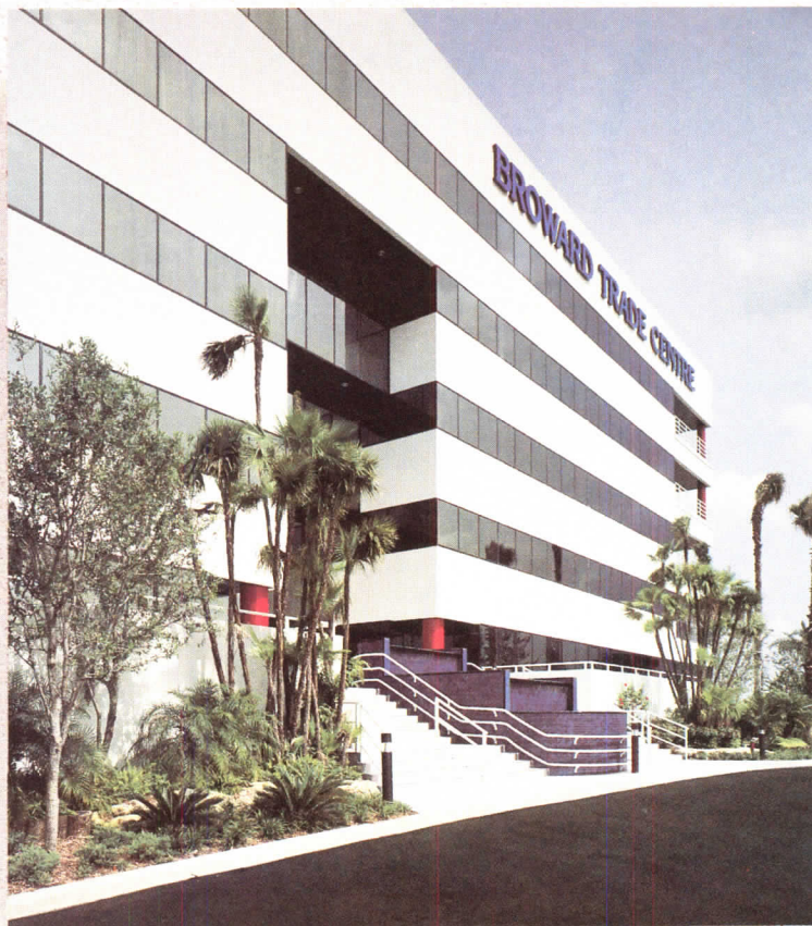
Broward Trade Center Fort Lauderdale, FL. Certified Applicator: RAMCO, Inc. General Contractor: Knight Enterprises
