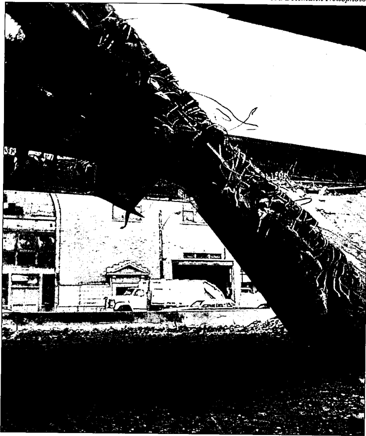
The gradual deterioration and ultimate collapse of the West Side Highway in Manhattan led to the initial proposals for Westway.
