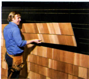
Install 8-feet of shingles in a shake.
