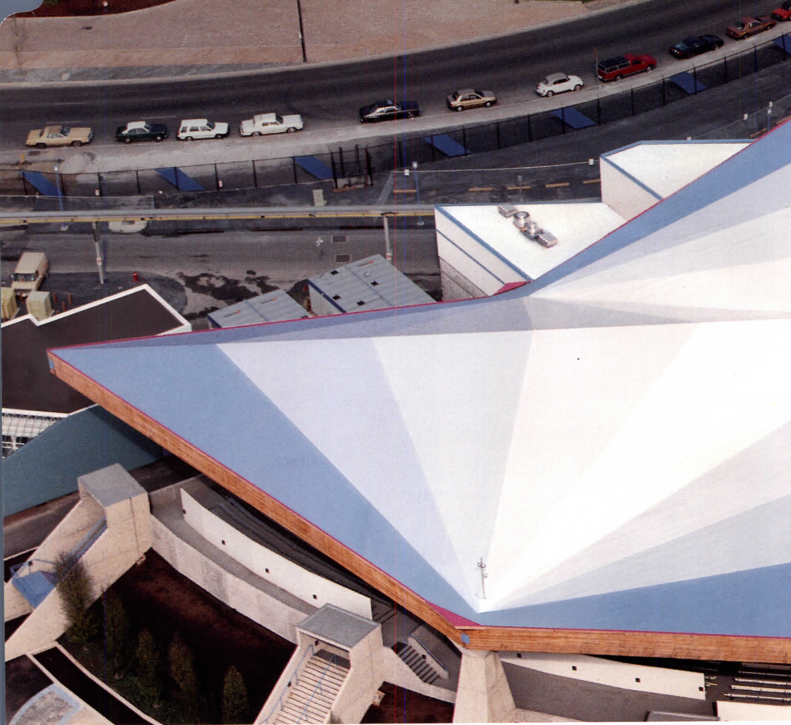
Building: Expo '86 Theater, Vancouver, Canada Architects: Aitken Smith Carter Partners; The Wade Williams Partner
