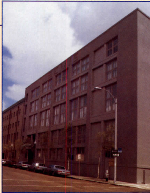
Bemis Bag Warehouse, built in 1906, is the first poured concrete building in Louisiana. Today it is Julia Place, 110 apartments located in downtown New Orleans. It's another historical building preserved by Alenco.
