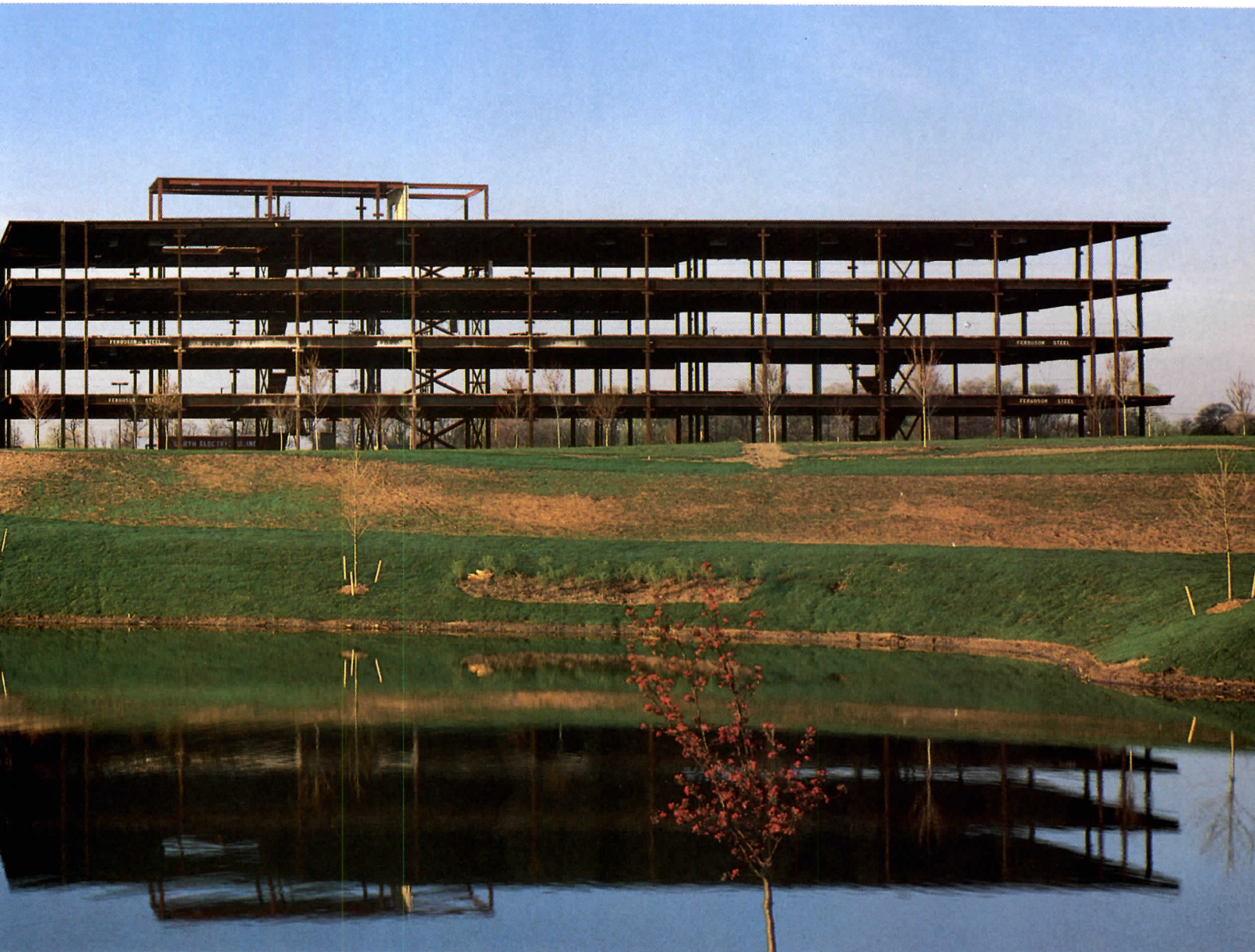
The Woodfield at The Crossing office complex in Indianapolis used 216 tons of Vulcraft joists and 169,000 sq. ft. of Vulcraft steel deck.
