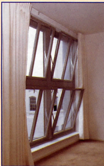
Exterior windows tilt in for easy cleaning. Heavy duty architectural windows with insulating glass preserve the historical feeling of this building.
