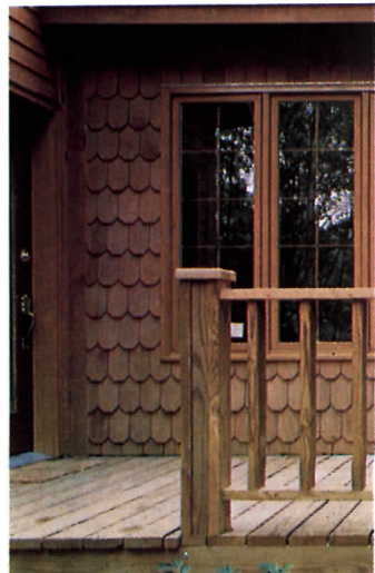
An entry treatment like this can open the door to a sale.
