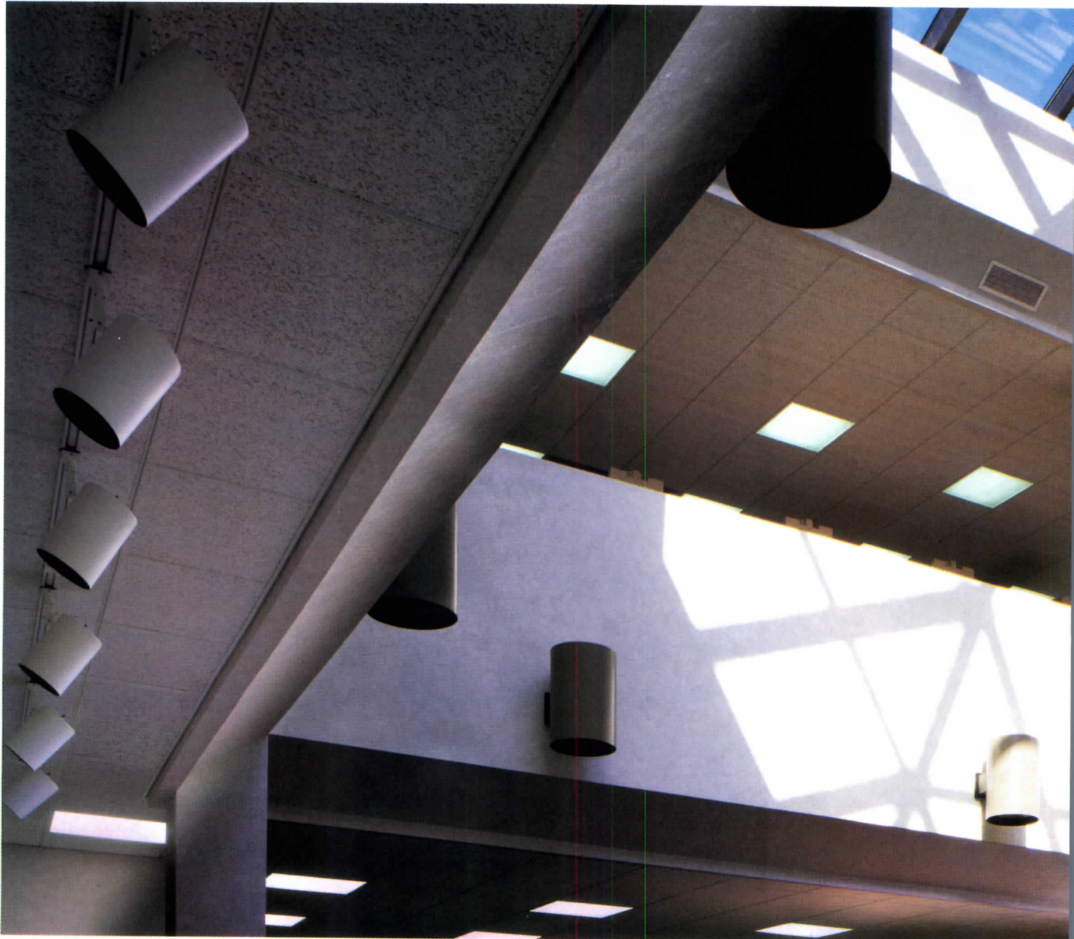
HANNIBAL FREE PUBLIC LIBRARY, HANNIBAL, MISSOURI ARCHITECT: JIM KREWSON, A.I.A. Spectra 3700 in white combined with standard white lay-in ceiling panels.
