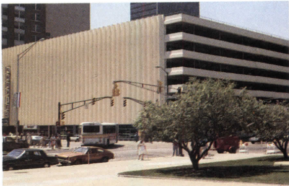
Dennison's Parking Garage, Indianapolis
