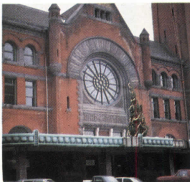
Union Station, Indianapolis
