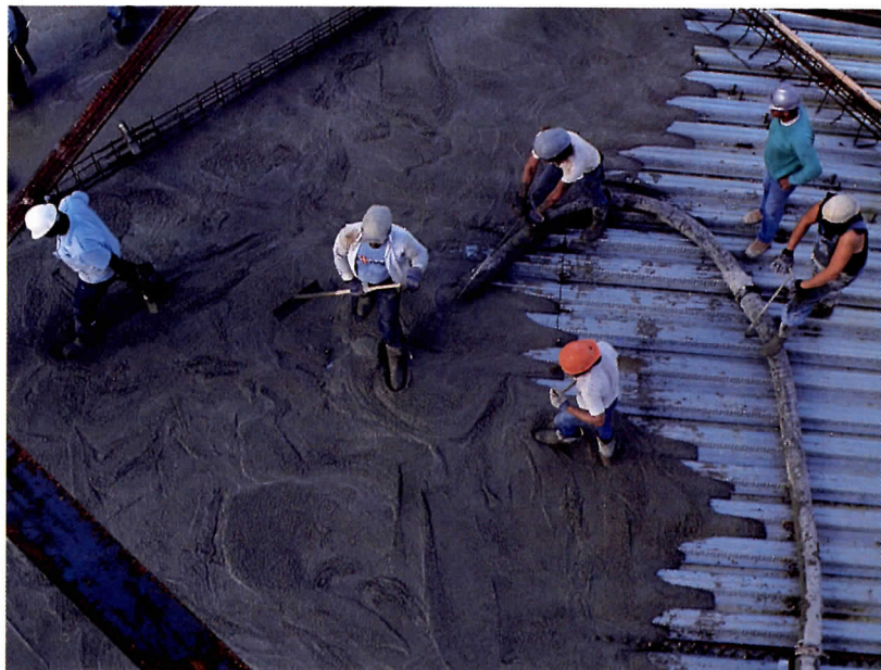
Installing Vulcraft composite deck is faster and more economical than poured-in-place concrete.
