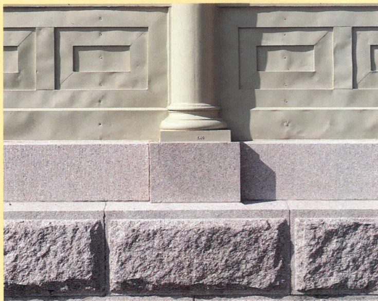
Cast-iron columns and panels were cleaned and repainted.
