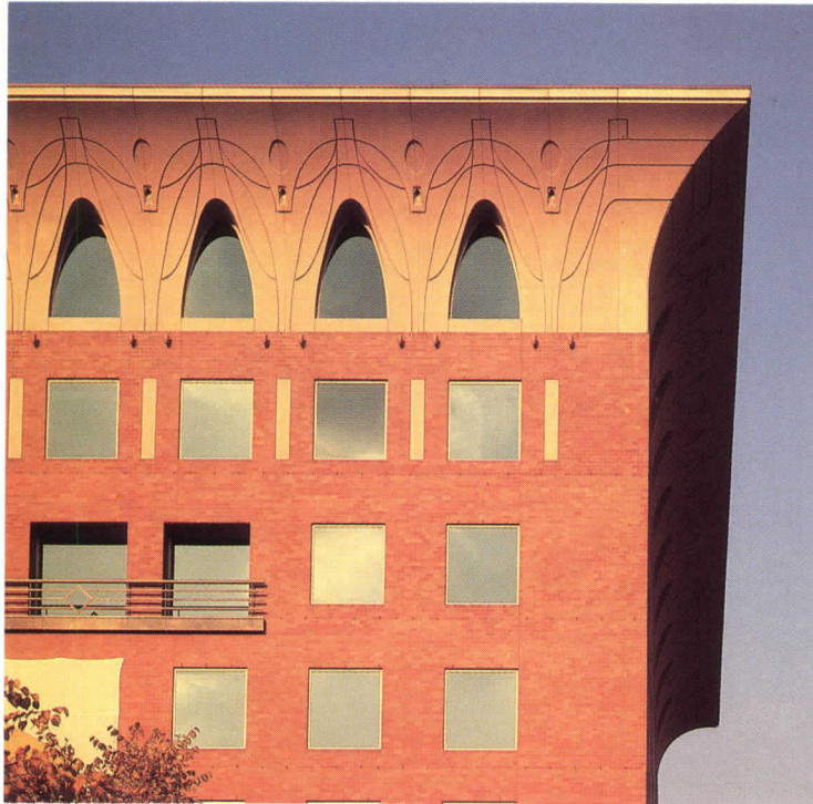
This stonelike cornice is glass-fiber reinforced concrete.
