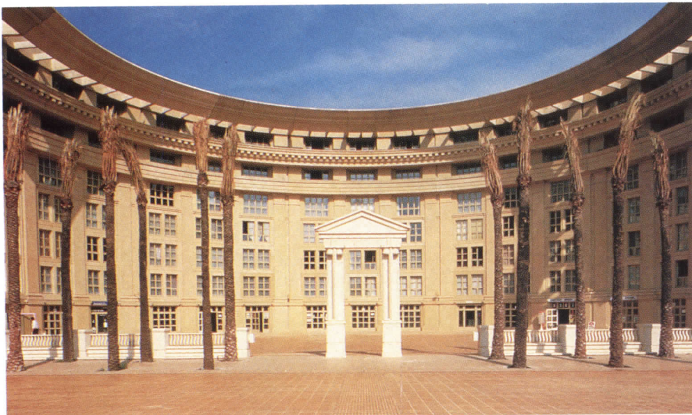
Antigone's site plan (top) reveals the project's axial organization, while its architecture (above) shows Bofill's love of baroque design.
