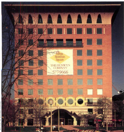
One Bowdoin Square's top-floor "cornice" is 39 panels of GFRC.
