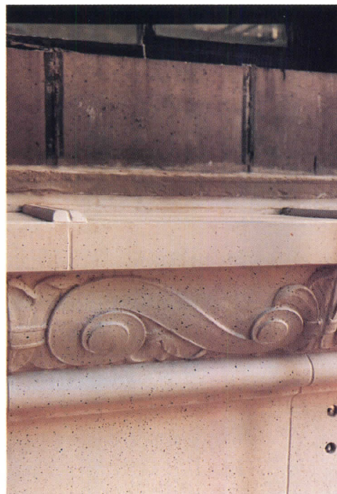
The gelcoat's color and pattern match the original terra-cotta cladding.
