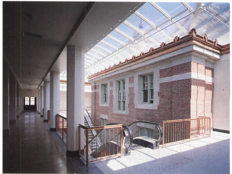
Exterior details have been restored indoors.
