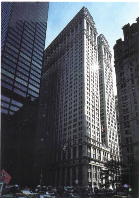
Drawings (right) were prepared from field surveys for remedial GFRP work at 120 Broadway (above).
