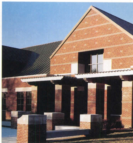
Imperatore Library, Englewood, New Jersey Architect: Bohlin Powell Larkin Cywinski Photo: Christopher Barone
