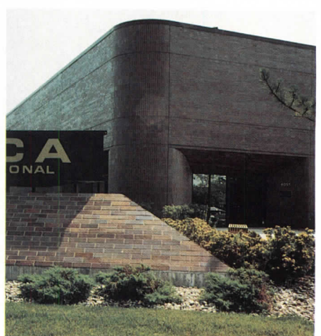
Building Officials & Code Administrators International, Inc., Flossmoor, Illinois Architect: Linden Group, Inc. Photo: Linden Group, Inc.
