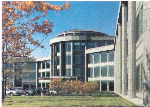
Disengaged exterior columns and flamed and honed granite cladding herald the rotunda interior.
