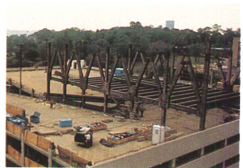
The Presbyterian-University Hospital Tower (middle) rises 21 stories. Installation of transfer trusses at the Biomedical Sciences Tower (above).
