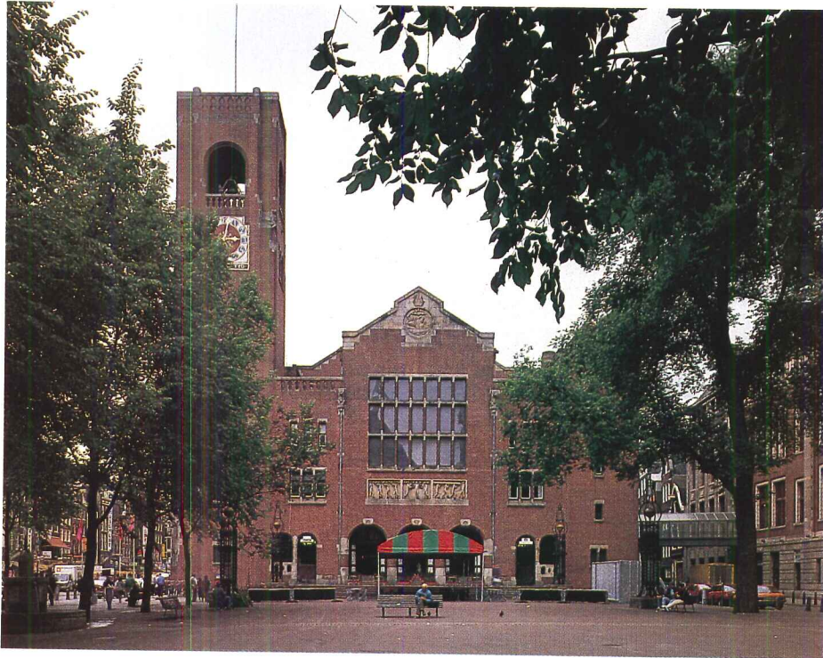
The south facade of Berlage's Exchange faces Beursplein Square.
