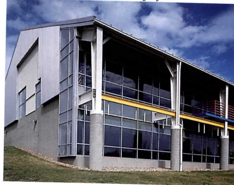
Top: The Pakatakan Industrial Park contrasts with an earlier method of systems building—a barn. Bottom: Pre-engineered framing is exposed at the Sheet Metal Workers' Union Hall.
