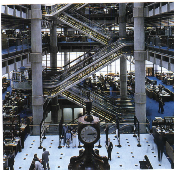
Richard Rogers's 1985 headquarters for Lloyd's is a 14-story glass shed that is hardly visible within a network of service pods containing stairs, elevators, and the vast mechanical infrastructure required by computer-intensive financial trading (9). It still ranks among the most sophisticated projects ever built in the way it integrates mechanical and other services into ceiling, raised access floor, and workstation. The sun-drenched 240-ft-high atrium (10) is oddly reminiscent of Wright's Larkin Building. With lush plantings, lounges, and eateries, Niels Torp's 1976 headquarters for
