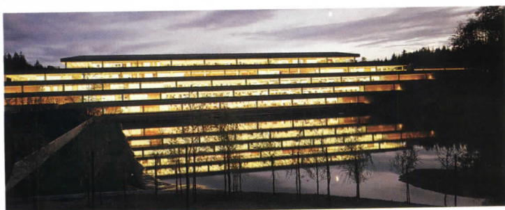
5 Skidmore, Owings & Merrill's headquarters for Weyerhaeuser, near Tacoma, Washington, used a long-span concrete structure and vast horizontal stretches of glass, broken only by silicone butt-glazing joints (5). Daylight pours into the floors. Nearly
