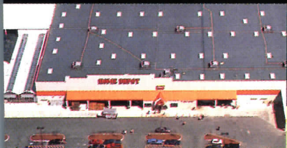
Hi-Tuff/EP works at Home Depot.
