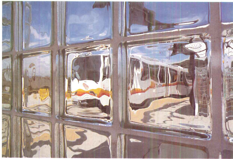
Regional Transit District Station • Denver, CO • Pittsburgh Corning's VISTABRIK® Solid Glass Block Jerry Cleveland, Photographer
