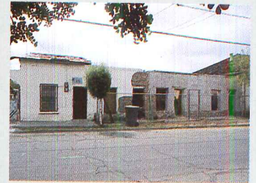
An old adobe wall (above) was restored as a freestanding entry (top) using traditional lime plaster. Existing openings were used for a new door, gate, and windows.
