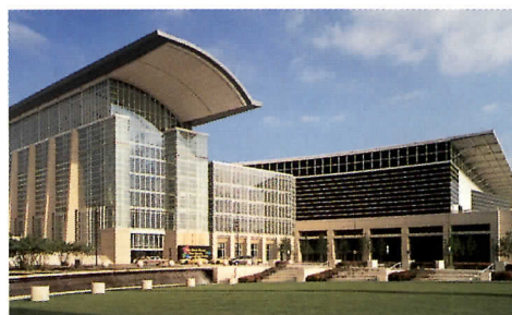
The Design Center in Linz, Austria, has a laminated glass roof that evokes crystal palaces (above). The expansion of McCormick Place in Chicago (left) is clad with low-e glass.
