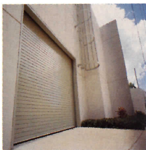
The Arecibo Observatory's operating facility includes an Atlas Door™ coiling steel service door.
