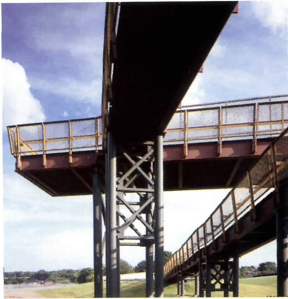
The New Street Pedestrian Bridge has a steel-grid deck with steel railings painted yellow (left). The jaunty buildings at the end of the Albany Street Bridge house restrooms and storage facilities (below).
