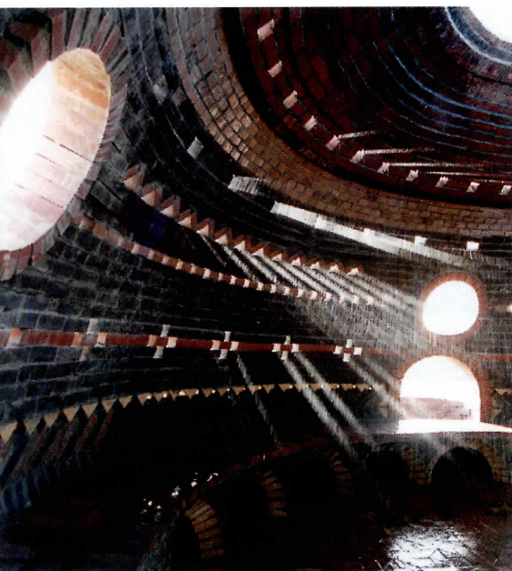
The Khalili-designed Rumi Dome (above), made of fired brick, and a superadobe structure (top).
