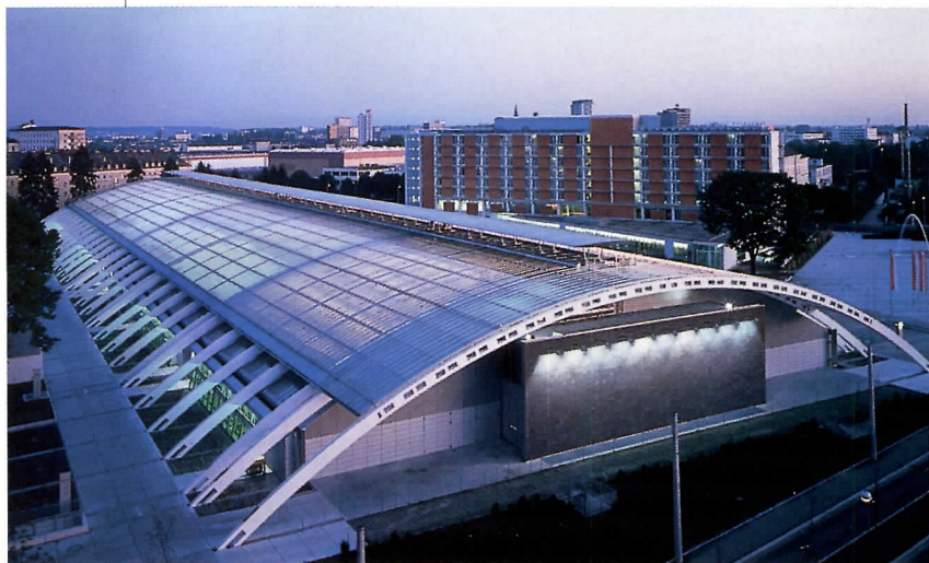
The Design Center in Linz, Austria, has a laminated glass roof that evokes crystal palaces (above). The expansion of McCormick Place in Chicago (left) is clad with low-e glass.
